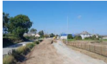
Footpath & Cycle lane Construction progress
