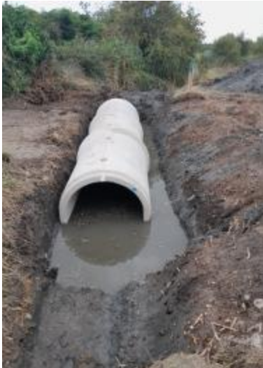
Commencement of pipe laying
