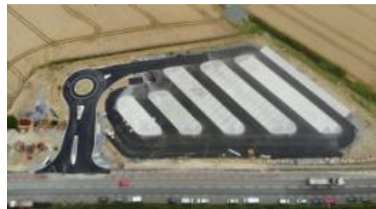
Aerial View of Park & Share Construction progress
