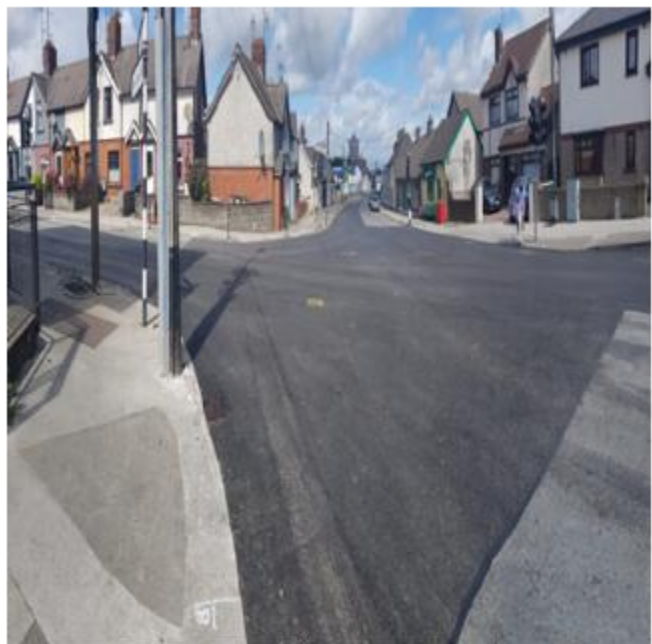
Platin Road/Beamore Road Junction Resurfaced
