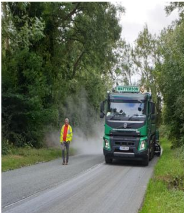
Surface Dressing on the R168 Collon to Tullyallen Road
