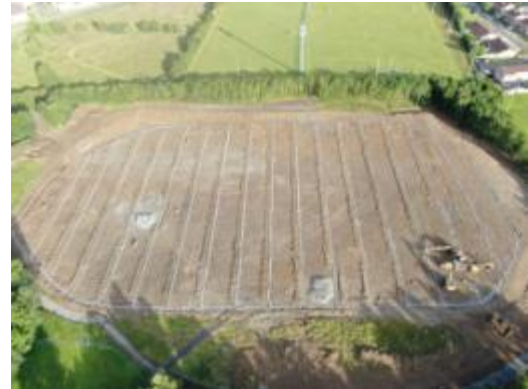
Aerial View of earthworks & drainage
