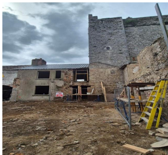
Demolition of Judges Chambers Completed
