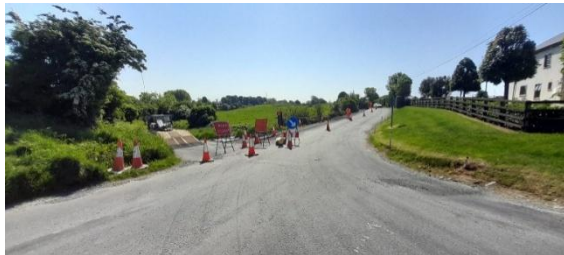
Vehicle Restraint Systems (VRS) works ongoing at Maguire's Cross, Cooley
