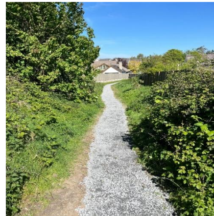
Pathway repairs completed at Green Lane, Blackrock
