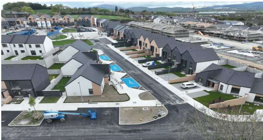
New Housing units at Fulacht Fia, Mount Avenue, Dundalk, Co. Louth
