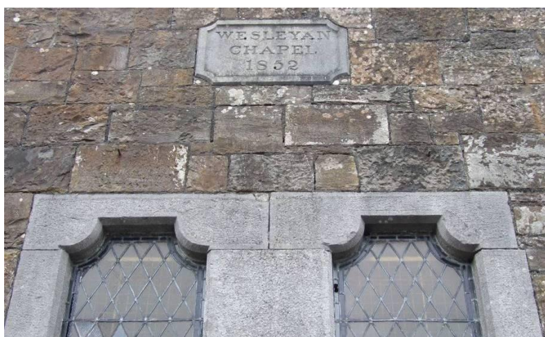
Fig. 109: Cut stonework to former Methodist Church
