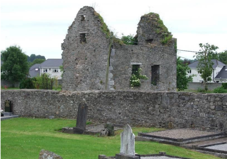
Fig. 96: View to Chantry College from St Mary's churchyard
