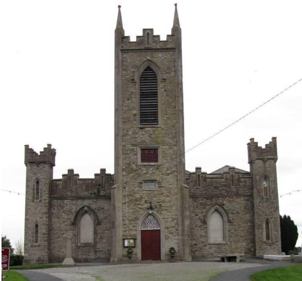
Fig. 47: Medieval Cross at St Mary’s Church
