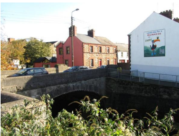
Fig. 59: Bridge seen from site of the former mill building
