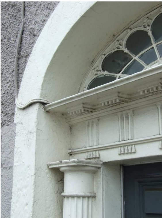
Fig. 103: Ionic detail to doorcase on William Street
