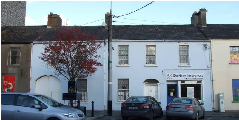
Fig. 24: Houses on east side of Castle Street
