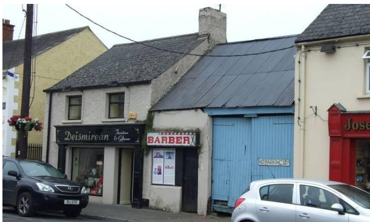
Fig. 122: Vernacular shop on Irish Street adds to the variety of the streetscape
