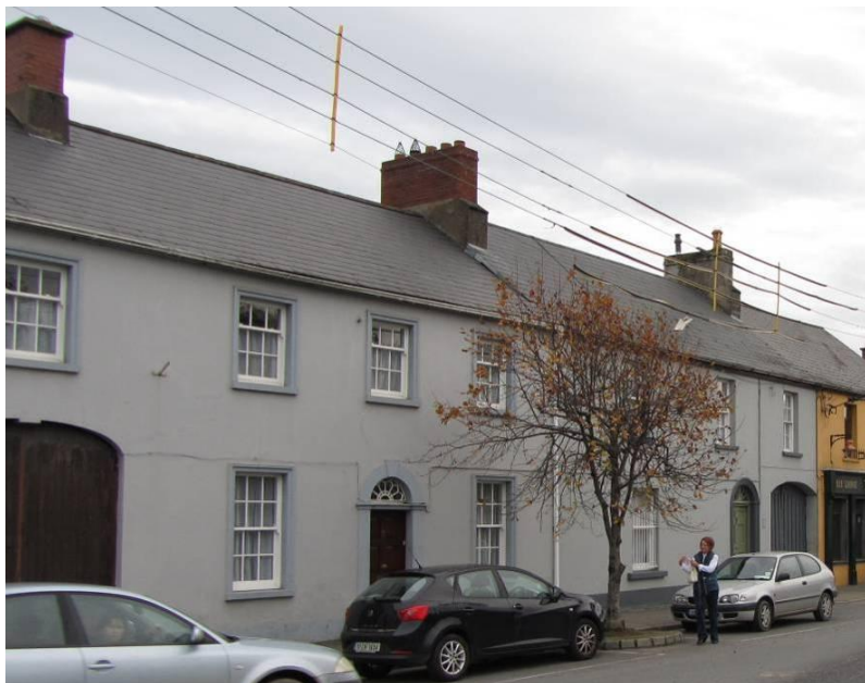
Fig. 23: Houses to east side of Irish Street
