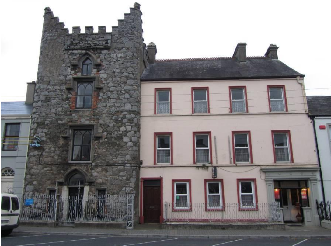
Fig. 51: Hatch's Castle, Market Street
