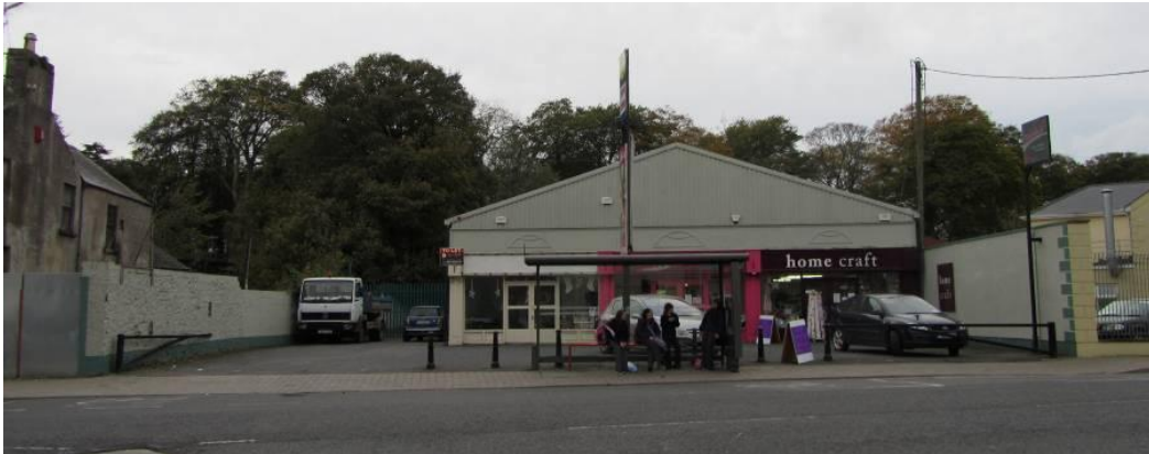
Fig. 130: New buildings which ignore the established building line and plot sizes damage the character of the street space
