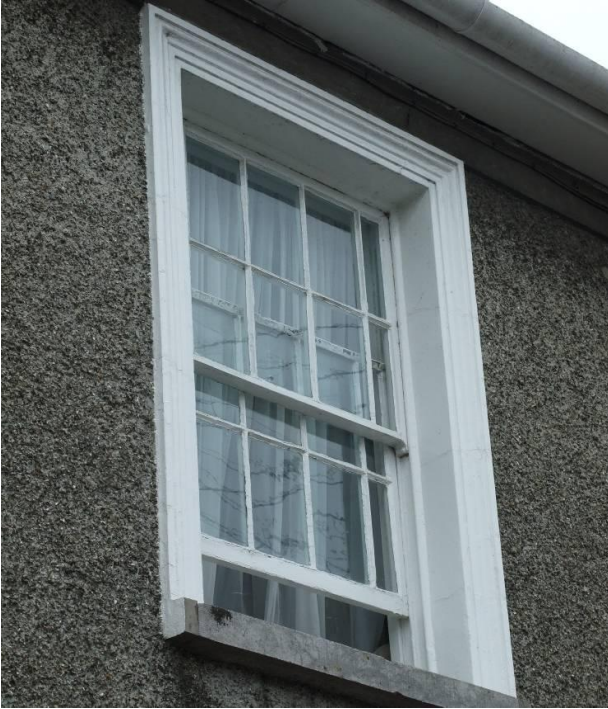
Fig. 117: Historic windows are perhaps the single most important element of an historic streetscape
