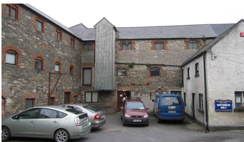
Fig. 62: Former dwelling to rear of Market Street
