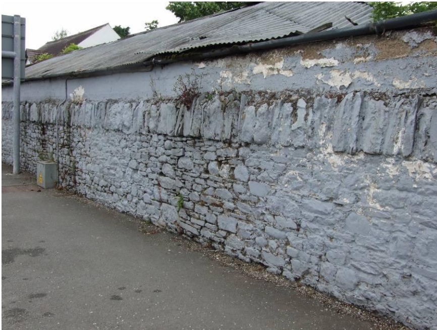
Fig. 104: Traditional stone masonry wall on Dundalk Road
