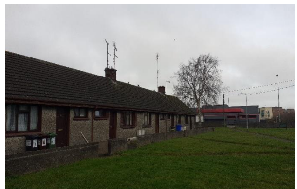
Ladywell Square, Dundalk, 1 st Properties to undergo Energy Efficiency works in 2025.
