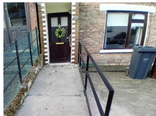
A ramp that was completed in December 2024, by an applicant who received a grant under the MAG scheme in Drogheda.
