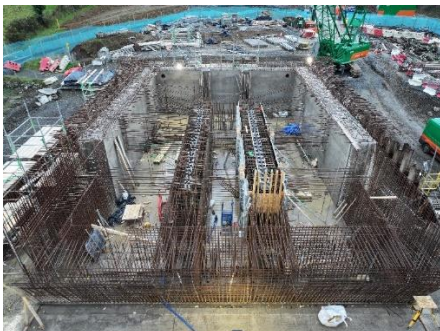
Southern Abutment ongoing R.C. works
