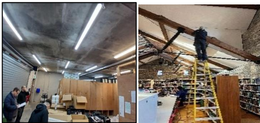
Lighting Upgrades at Ardee Civic Centre & at Dundalk Bookstore
