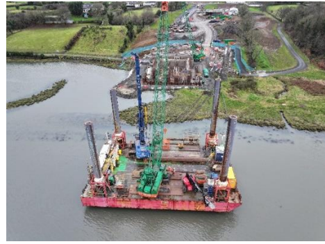
Marine Piling Works
