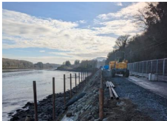
Substructure substantially complete between Rough Island and Victoria Lock
