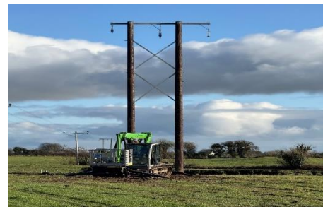
High Voltage ESB Network Diversion
