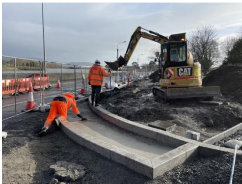
Works ongoing (Phases C, F and E)
