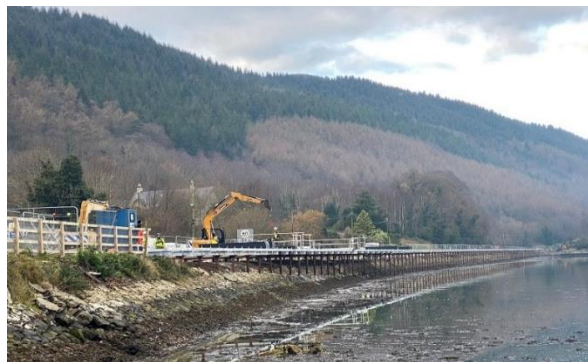
Substructures complete between border and Rough Island
