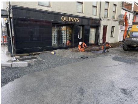
Works ongoing to Bridge St. (Phase B LHS)
