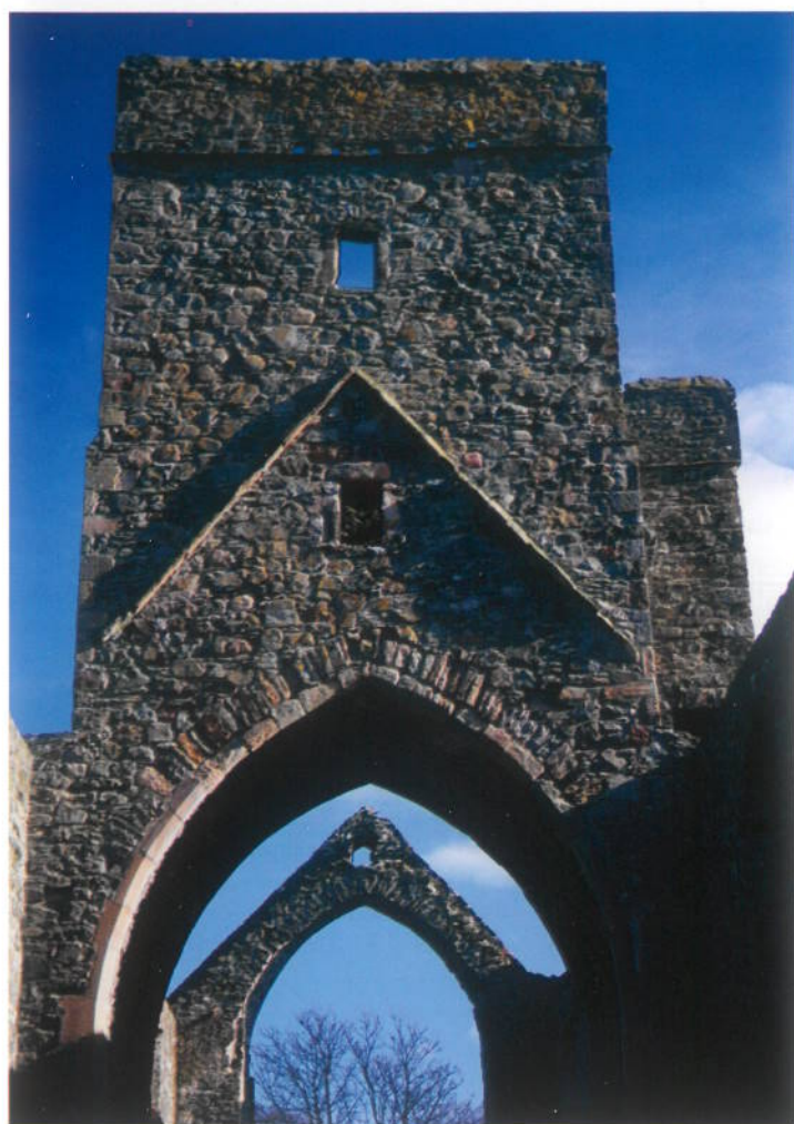
Top: View of the south wall of the church, showing large flat-headed window and doorways leading to nave and chancel. The external string-course along the western portion of the south wall marks the position of the cloister roof. The gable lines of the east range can be seen to the right of the south wall.
