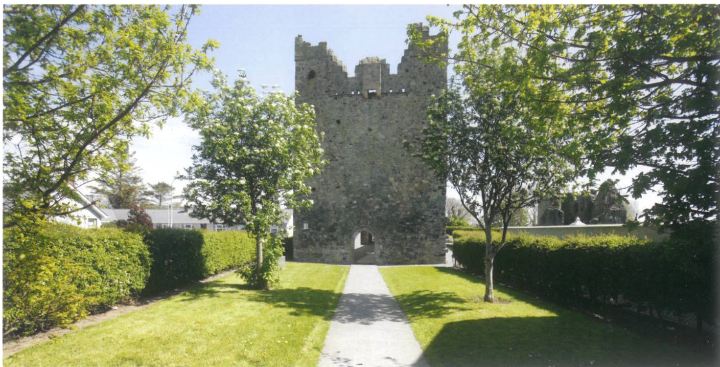
Below: View of fortified portion of the nave, showing the crenellated west wall, a machicolation above the arched doorway and the added corner towers.
