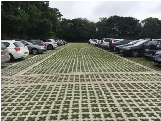
REINFORCED GRASS SYSTEM RV Parking Area
