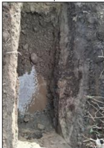
INFILTRATION TEST - PHOTOS
