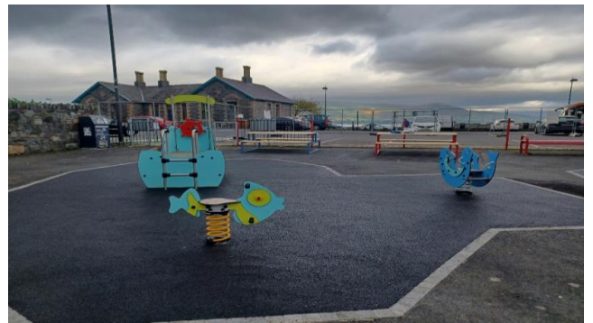
Newly refurbished Playground in Carlingford
