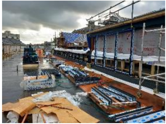
Block N New Link Building : Window Installation
