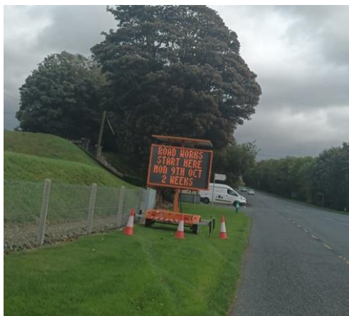
Roadworks at Monksland
