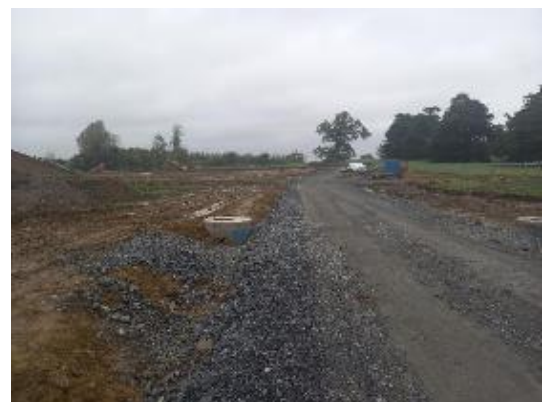
Site Clearance for the school site on the left
