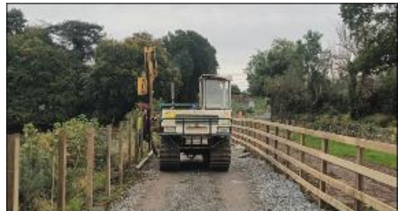
Permanent Fencing installation Cornamucklagh
