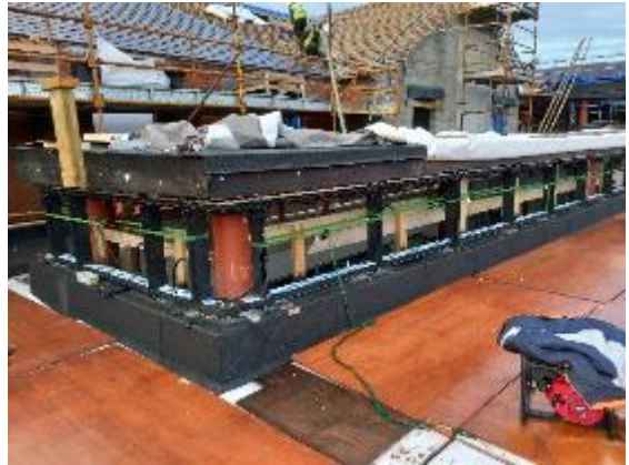
Block N New Link Building : Window Installation
