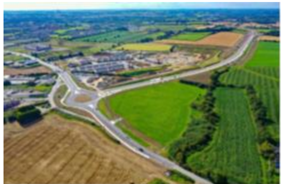
Ballymakenny Roundabout looking west
