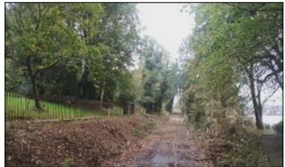
Site clearance through Omra Park
