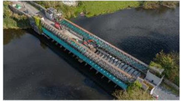
Drone footage of deck removal
