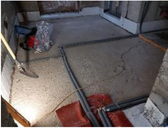
Block C Lift Hallway Floors pre screed pour, all now completed.
