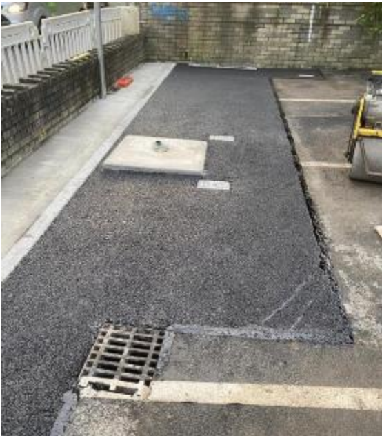
Civil Works underway Donore Rd Car-Park Drogheda
