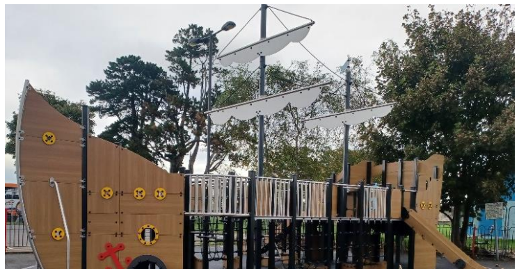
Refurbished Playground at Carlingford
