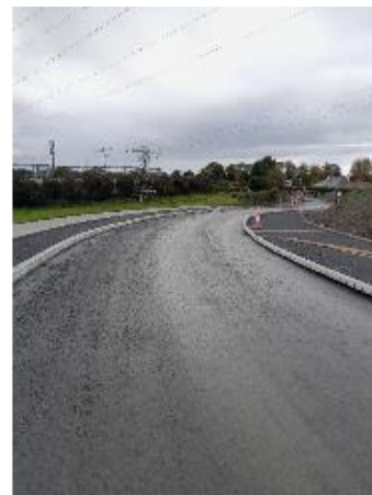
Road section with Cycle lanes and footpaths
