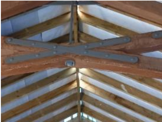
Block C Truss Ironmongery Treatment
