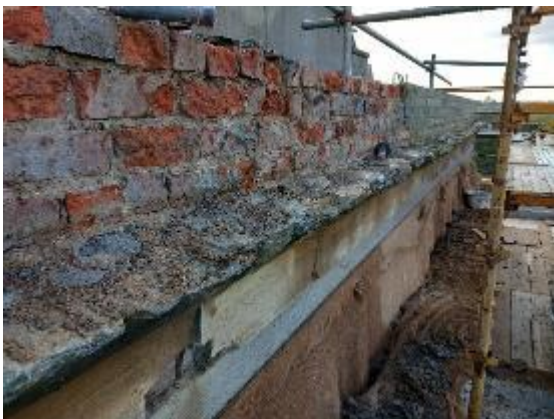
Block E Annex Building : Parapet Conservation Works
