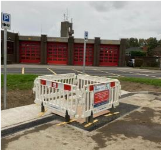
Ground works completed Dundalk (Tennis Club) Car-park
