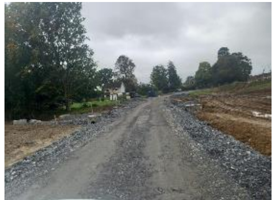
Access Road Construction
