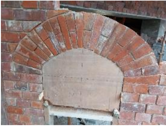
Block B rebuilt Brick Arch South Elevation
