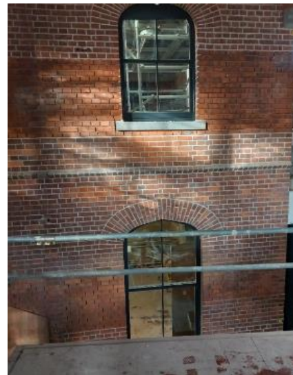
Refurbished Sash Windows East Elevation
