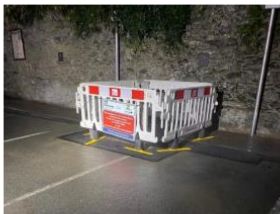
Ground works completed Ardee Car-park
