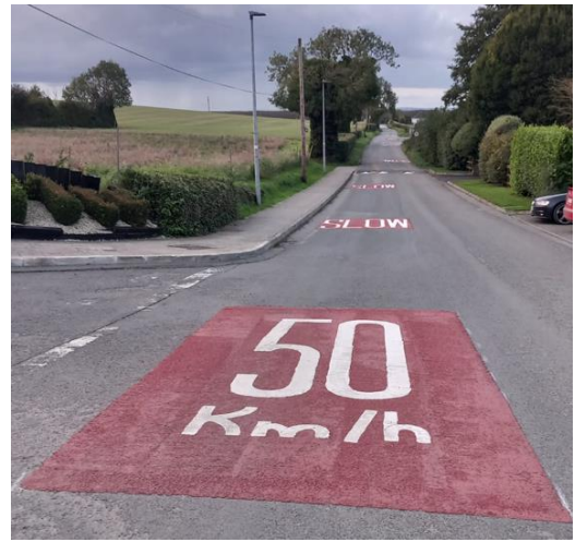
New road markings at Stabannon
