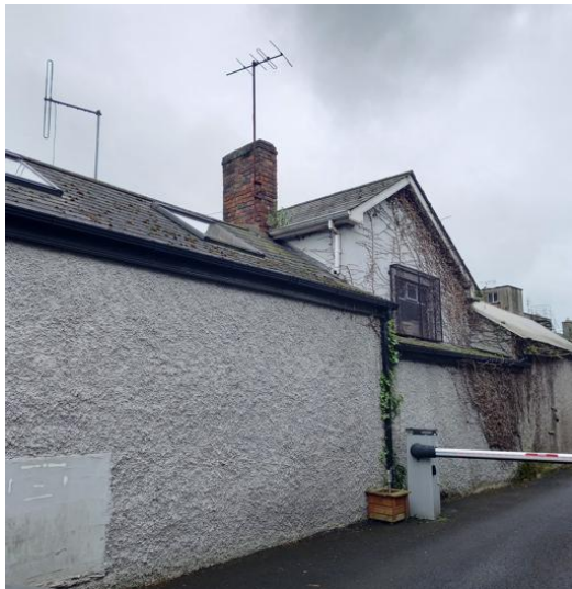
Above: Chimney subject of this section declaration.
