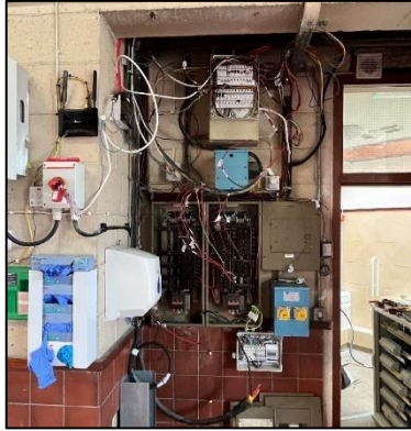
Photo: Sub Distribution Board Work Progress
