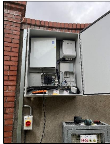
Photo: New Electrical Supply for Automatic Gates
