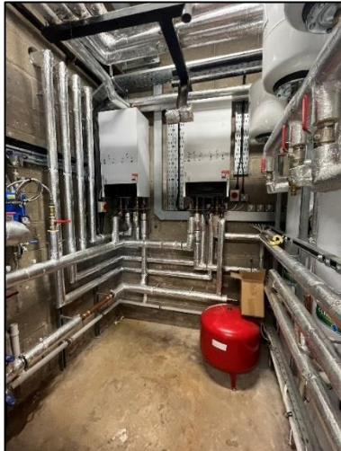
Photo: Dundalk Fire Station's Plantroom Progress
