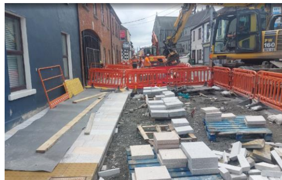
Linenhall Street, installation of new footpath ongoing.
