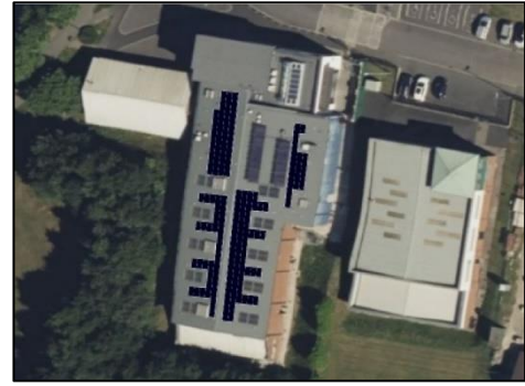
Photo: SPV proposal for a 138 x 435Watt Panel, 60kWp array, proposed for Muirhevnamor Sports Centre, Dundalk as part of a package of SPVs for 22 Council Facilities.
