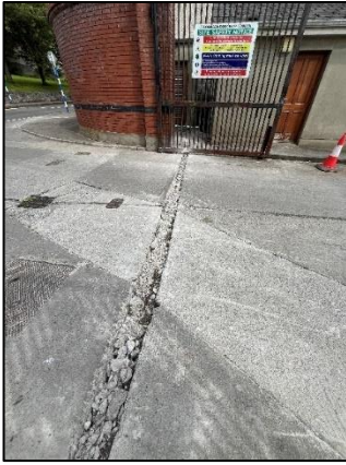
Photo: Cutting of Tracks for Ducting
