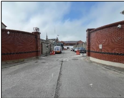
Photo: Drogheda Machinery Yard Gates Removed
