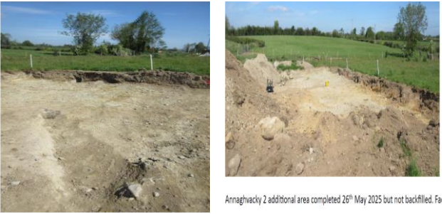
Annaghvackey 2 additional area completed 26 th May 2025 but not backfilled. Facing W.
