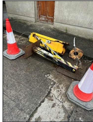
Photo: Removal of Old Barrier Equipment
