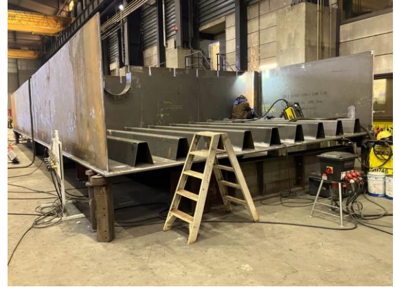
Commencement of Fabrication of Bridge Components
