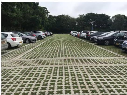
REINFORCED GRASS SYSTEM RV Parking Area
