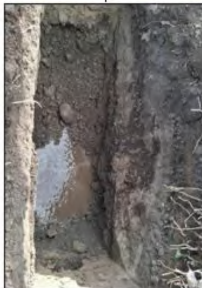
INFILTRATION TEST - PHOTOS
