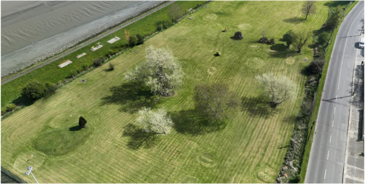
Figure 1: UAV Aerial Photograph of Site Facing Northeast at 60m Elevation
