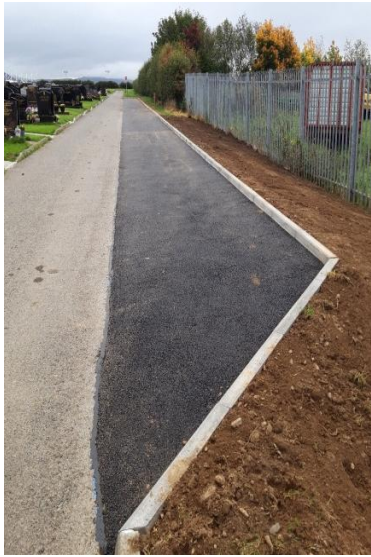
Grave-yard Lay-by installation Castlebellingham
