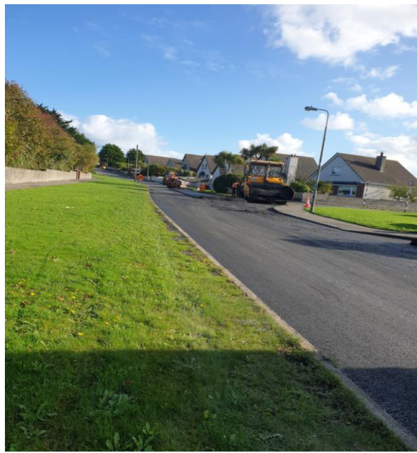
Resurfacing on the R166 Clogherhead
