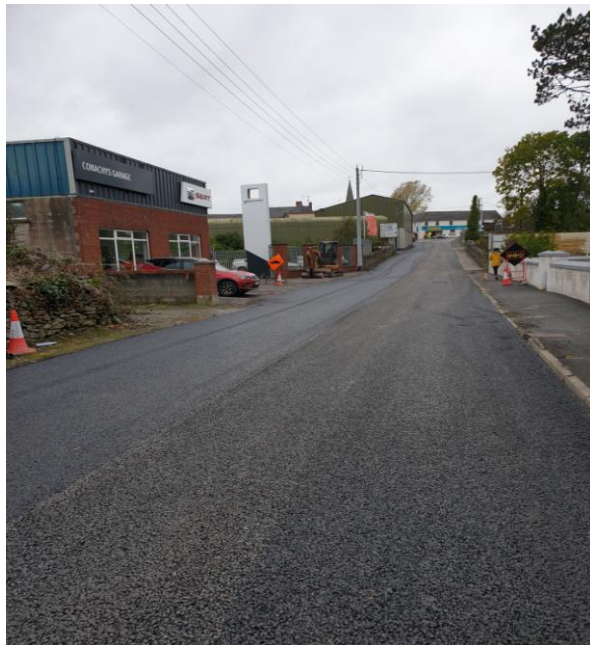
Resurfacing on the R170 Barn Road Dunleer
