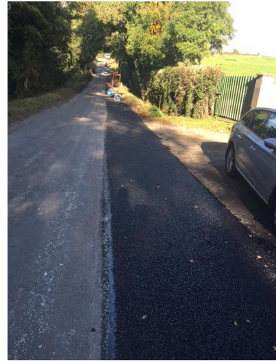
Edge repairs on the LP1264 Smarmore
