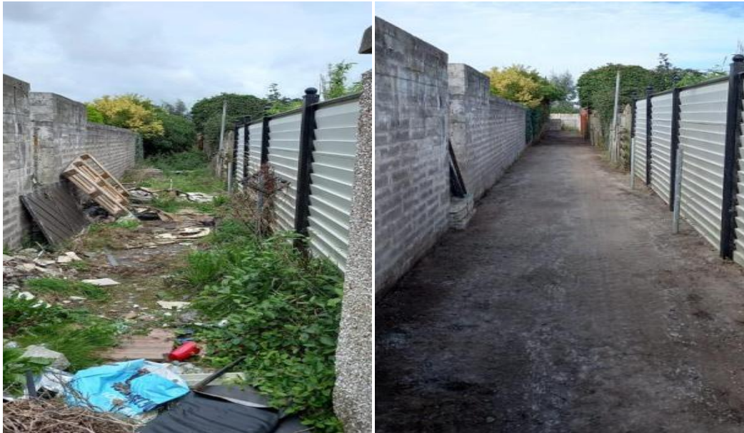
Clean up on back alley Marley Court, Drogheda
