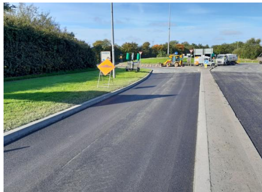
Laying of new road surface
