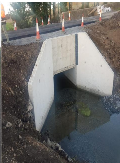
Works at Darver Bridge
