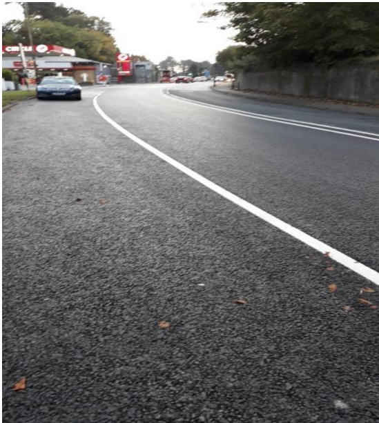
Resurfacing on Dublin Road Drogheda
