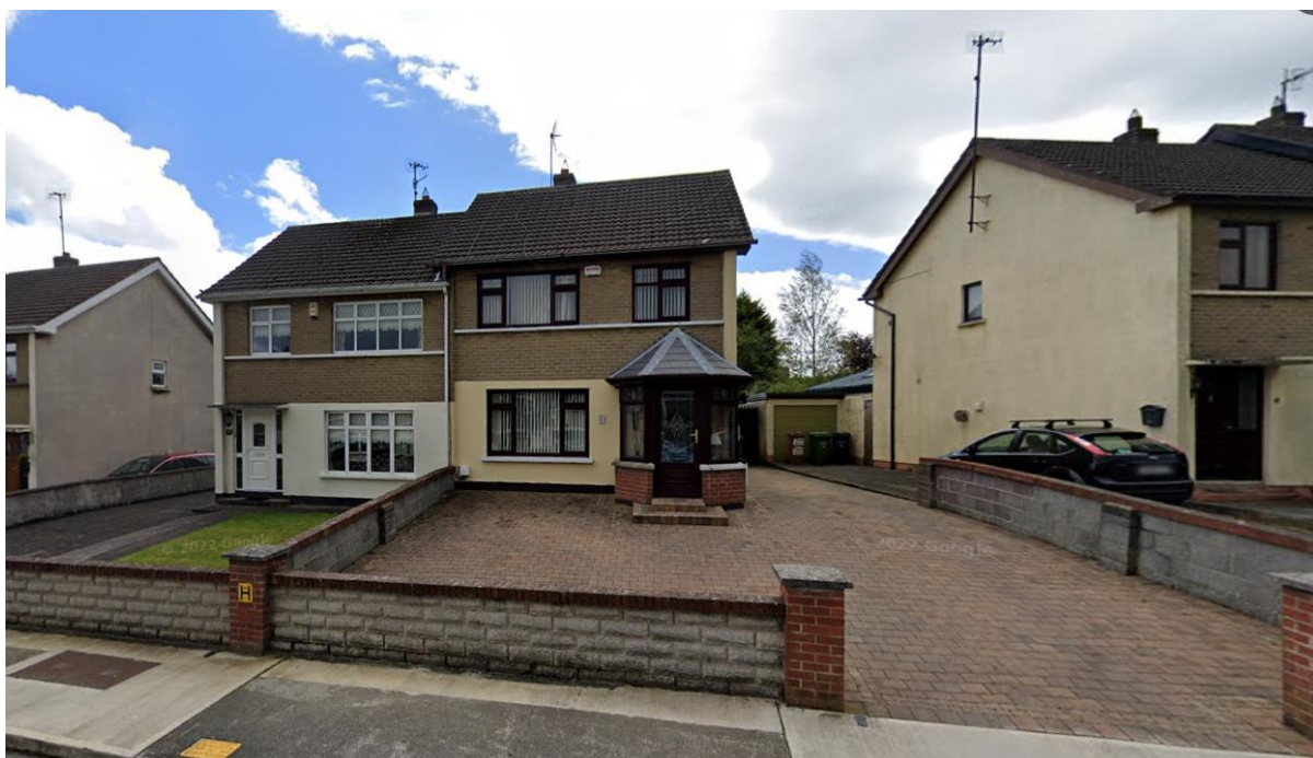
Fig.2: Existing dwelling (Google Streetview, May 2019)
