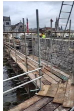
St. Dominick's Bridge- Wing-wall rebuilt
