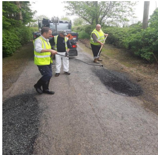
Pothole repairs at Bog Road Rassin LS7118-0
