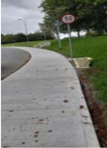
Footpath works completed in Cherrybrook Ardee
