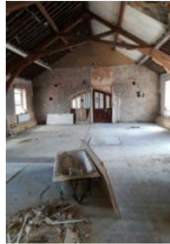
Community Services Building – stripping out underway
