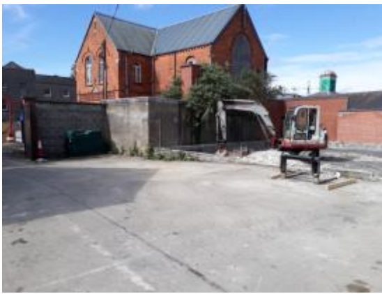
Demolition and removal of Old Glass Houses
