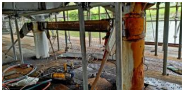
Structural Steel Columns under repair
