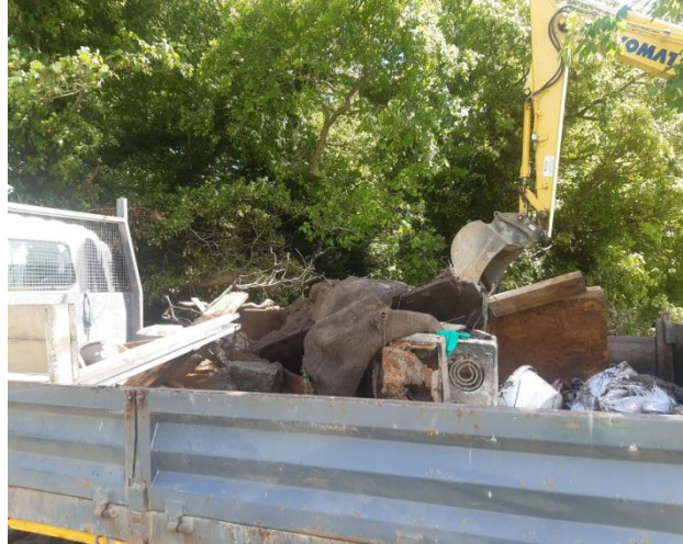
Flytipping at L2307, Greenhills
