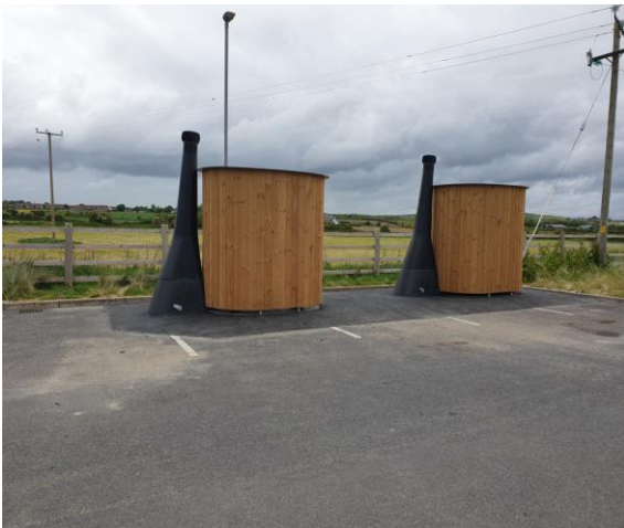
2no. Ecoloo's have been constructed at Seapoint Carpark, Termonfeckin. Ecoloo's are independent of water, sewer and electricity connection
