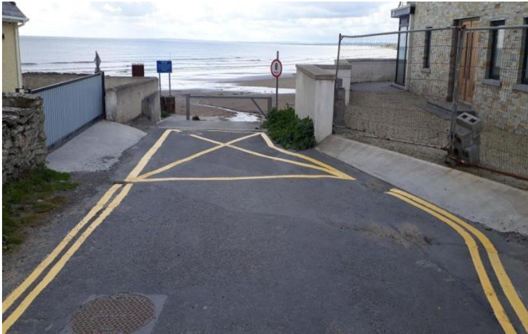
Photos above show new line marking at Crooked Street, Clogherhead
