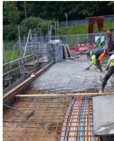
Reinforced concrete deck being poured
