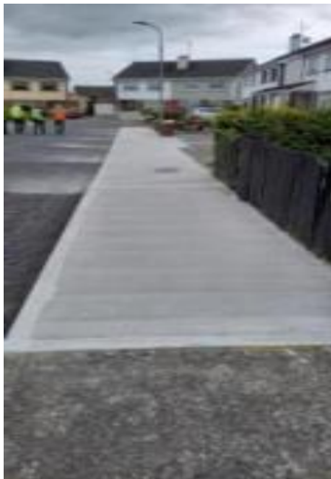
Footpath works completed in Cherrybrook Ardee
