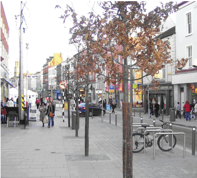
West Street Environmental Improvement Scheme
