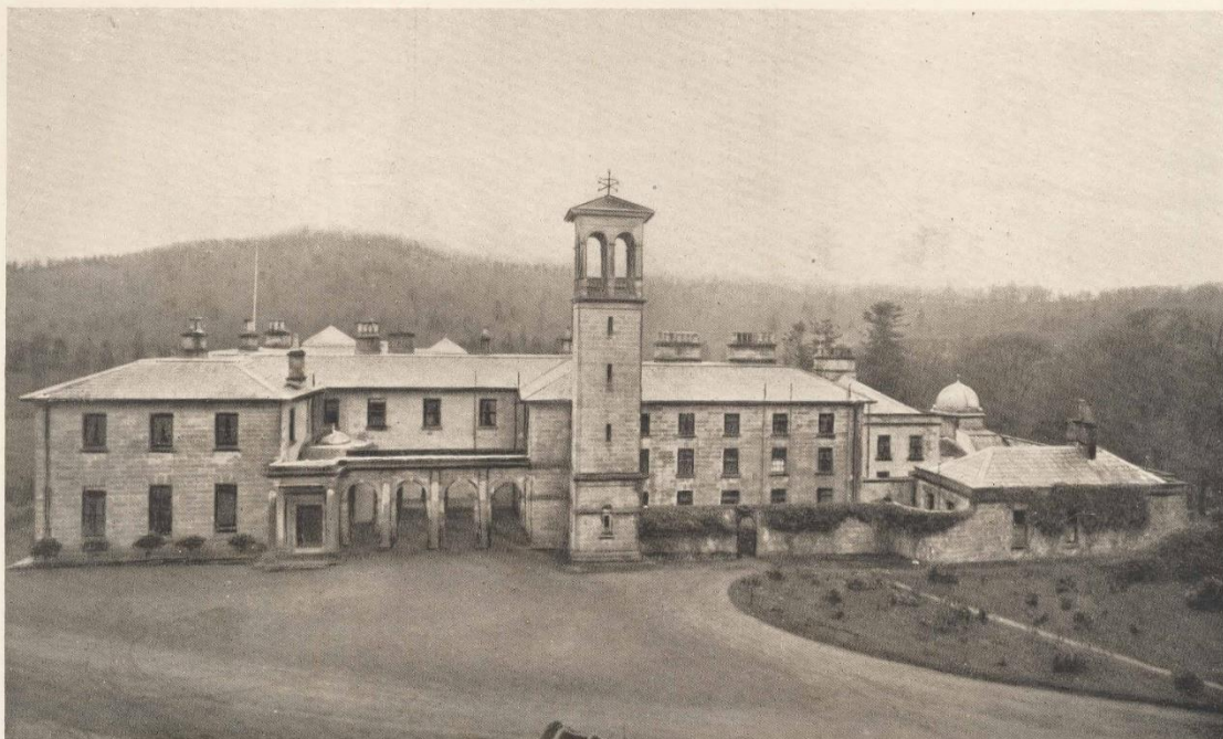
RAVENSDALE HOUSE (Front View).
