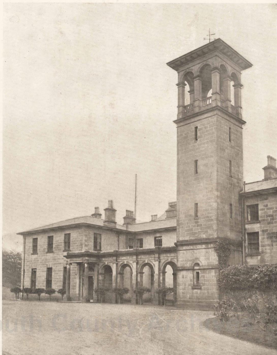
RAVENSDALE HOUSE.—ENTRANCE AND TOWER.
