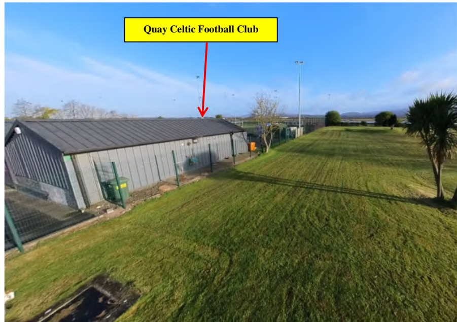
Plate 7. Ground panoramic photograph at the western boundary of the site facing in a north-westerly direction.
