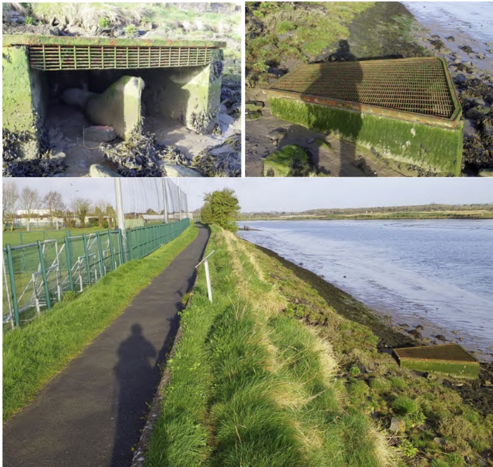
Plate 21. Various ground photographs of the Stormwater Outfall on foreshore to the north of Quay Celtic F.C.
