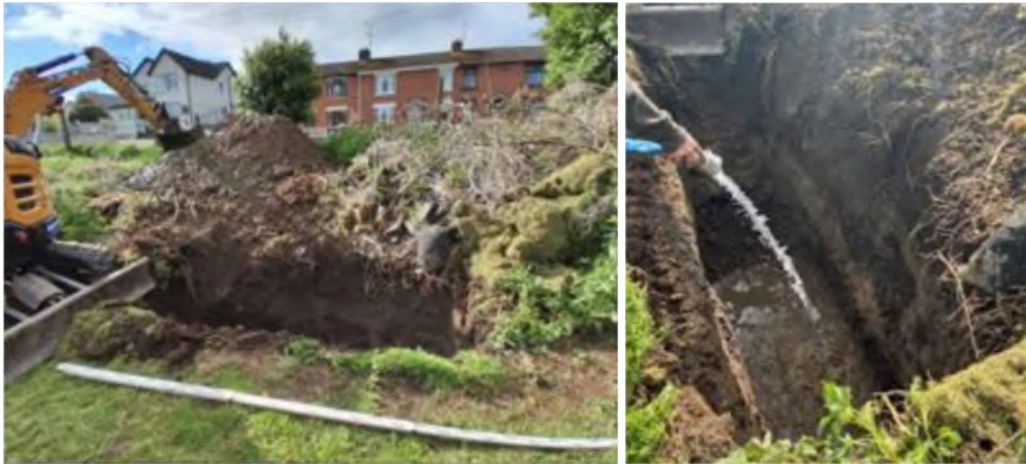
Plate 22. Ground photographs of trialpitting and BRE365 testing carried out to the south of the pitch and putt course to determine the suitability for a SuDS system
