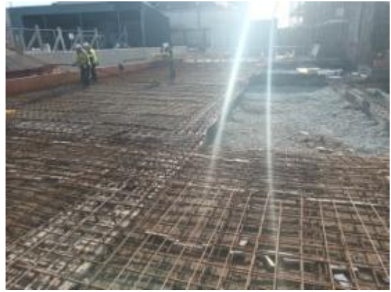
Block N New Link Building- Sub floor steel
