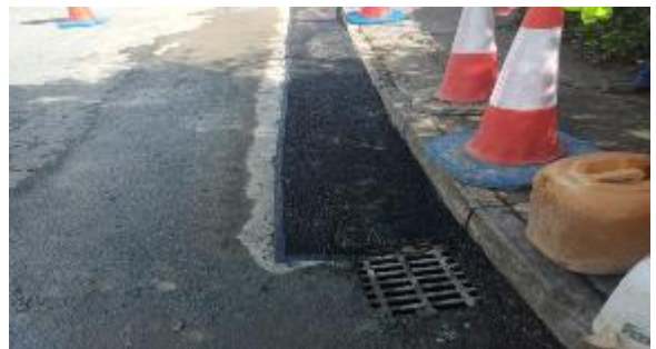
Repairs on the LP 2290 Collon to Tinure
