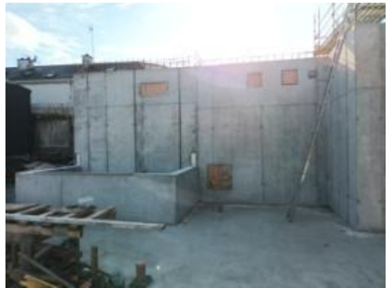
Block N New Link Building ESB substation Walls
