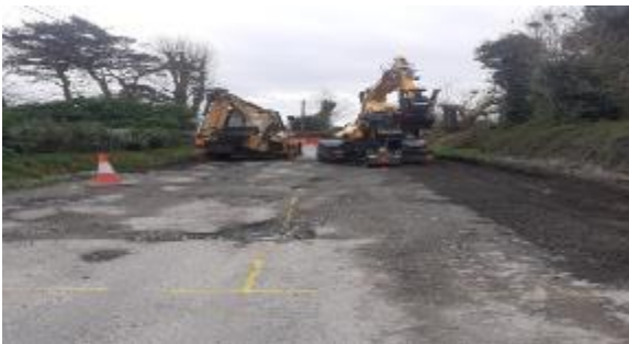
Ongoing works at Newtownstalaban
