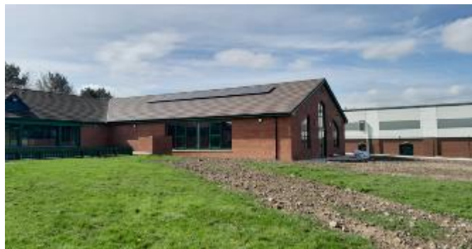
Muirhevnámór Community Centre Extension near completion
