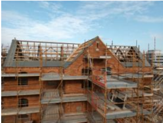
Block B Council Chamber Building – Temporary Roof Removal
