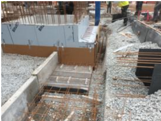
Block C Community Services Building- Lift base
