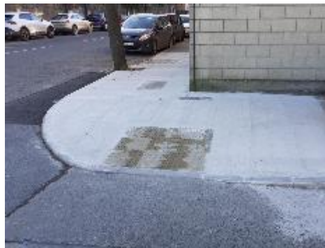
Footpath accessibility works completed at Castle Road
