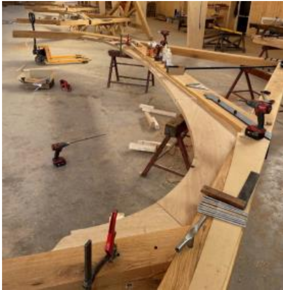
Block B trusses in production
