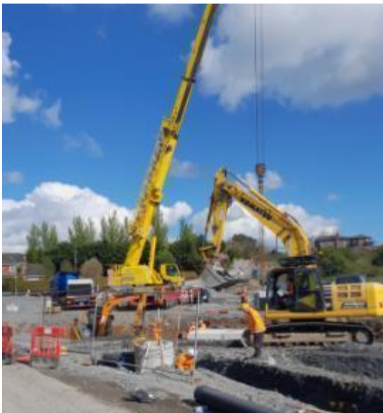
Culvert installation at Roundabout Location
