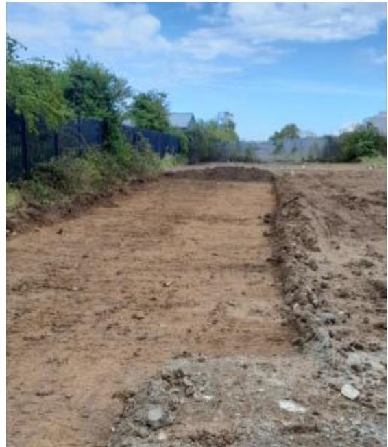
Topsoil Strip
