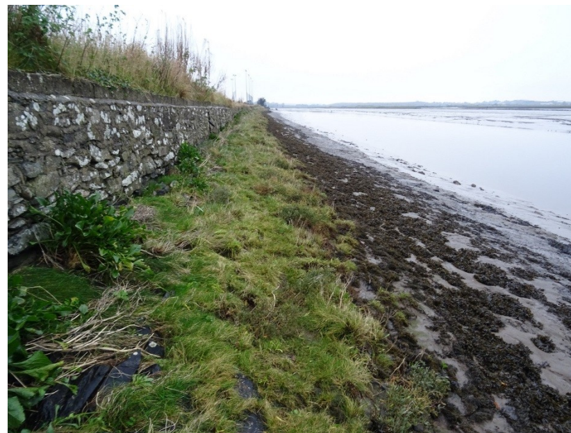
Plate 6: Stone wall along riverbank, looking west
