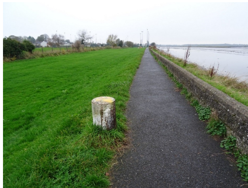
Plate 2: View of the north part of site, looking west
