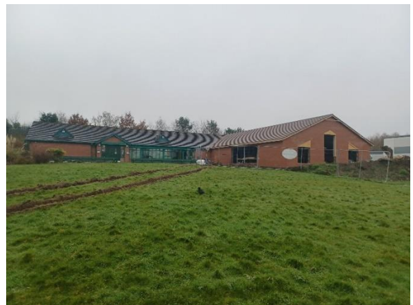
Progress of the extension at the Muirhevnamór Community Centre
