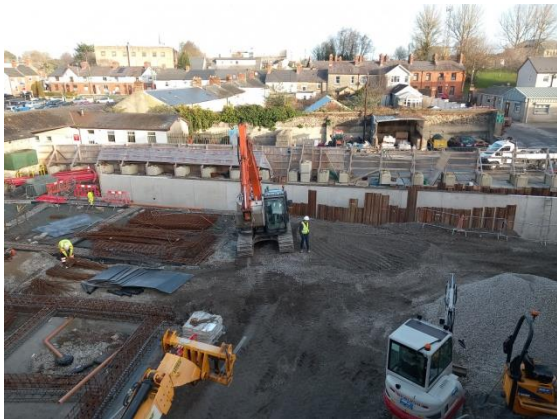
Northern Retaining Wall & Ground Beam fabrication Block N
