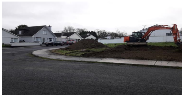
Site clearance works for new housing unit - School Lane, Dunleer
