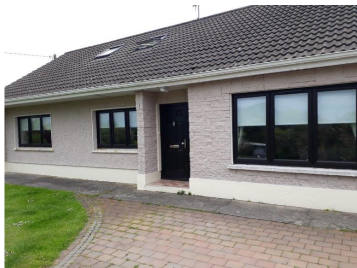
New Windows and Door funded by a housing adaptation grant in 2022
