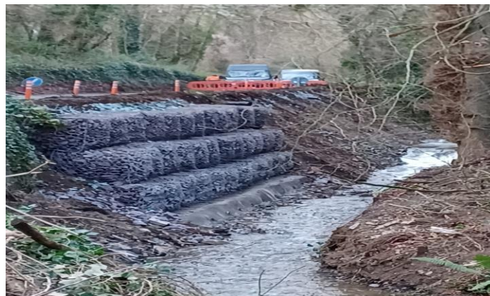
King Williams Glen Slope Stabilisation – new gabions installed
