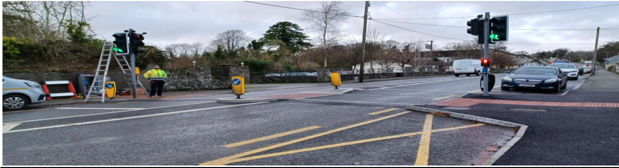
Traffic lights installation at Collon, Co. Louth
