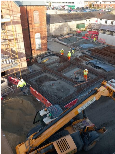
Ground Beams fabrication Block N –New Link Building
