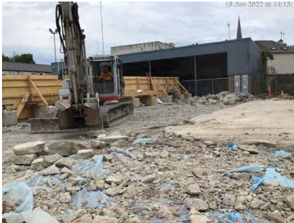
Breaking out of Concrete Maintenance Yard
