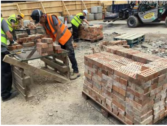
Cleaning of dismantled brickwork from Valhalla Building
