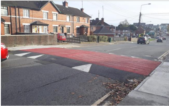
Hardmans Gardens Drogheda Raised Crossing
