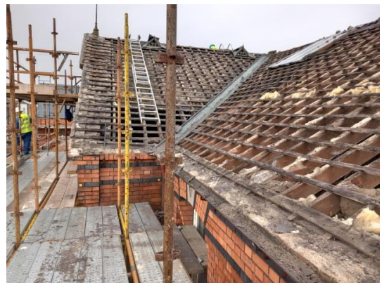
Roof dismantling Block Community Services Building
