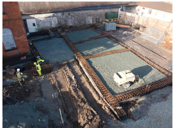
Ground Beam Construction New Link Building Block N
