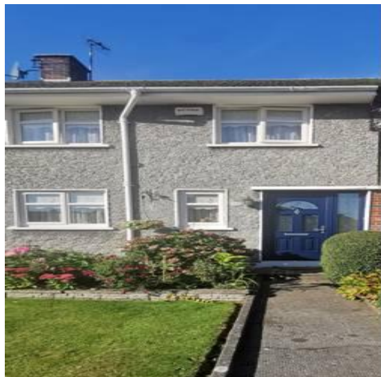
Housing For Older People New Windows and Door, Yellowbatter, Drogheda
