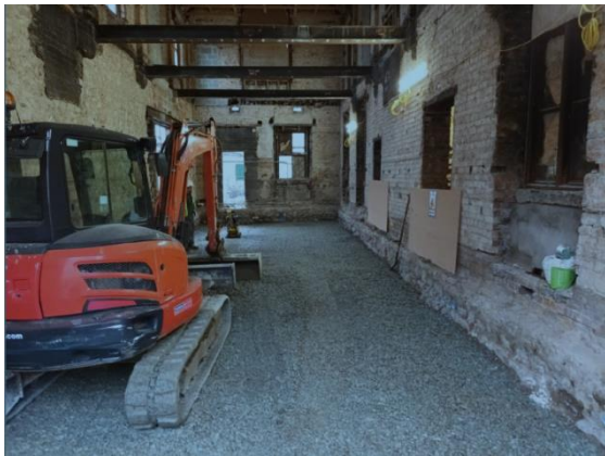
Fill in Subfloor Block B
