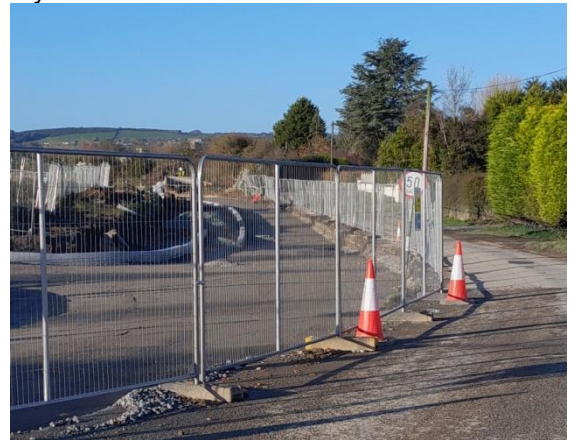
Works ongoing on the Twenties Lane realignment at DIFE
