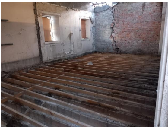
Floor stripping Block Community Services Building
