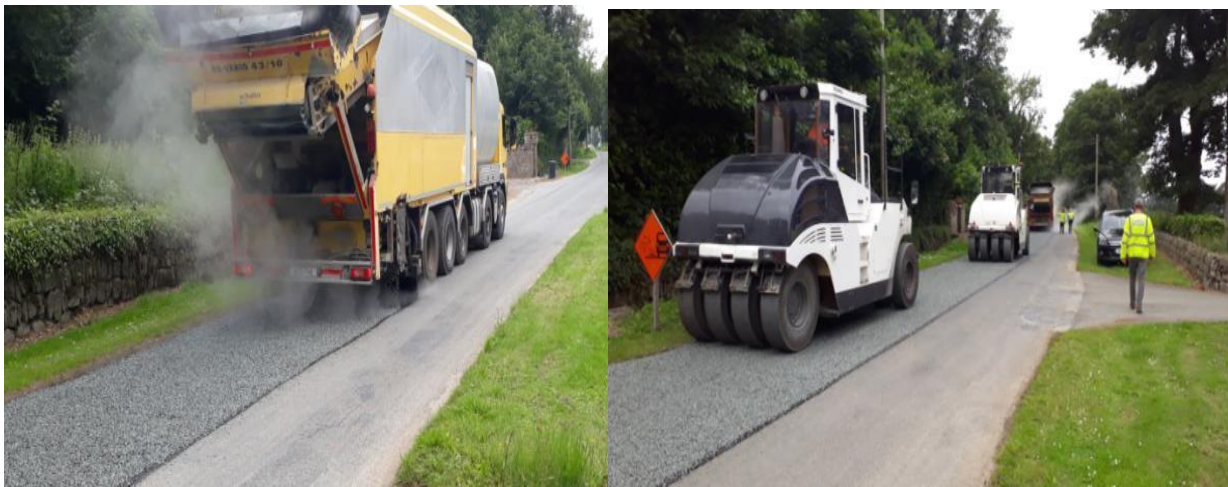
Surface Dressing at Richardstown
