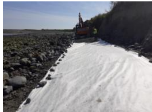
Haul Road to protect the SPC
