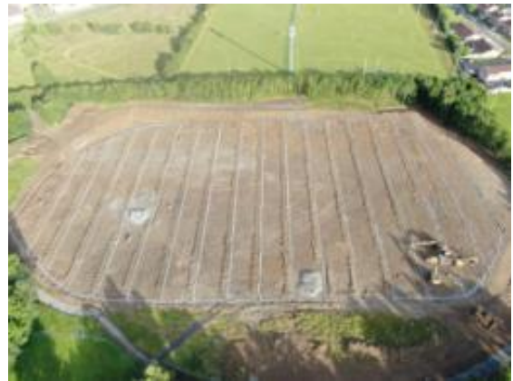
Aerial View of earthworks & drainage
