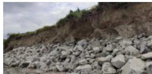
Rock Armour Works
