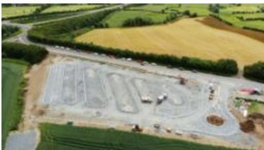
Aerial View of Park & Share Construction progress
