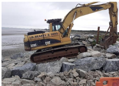
Figure 3 – Coastal Erosion Protection Works at Salterstown
