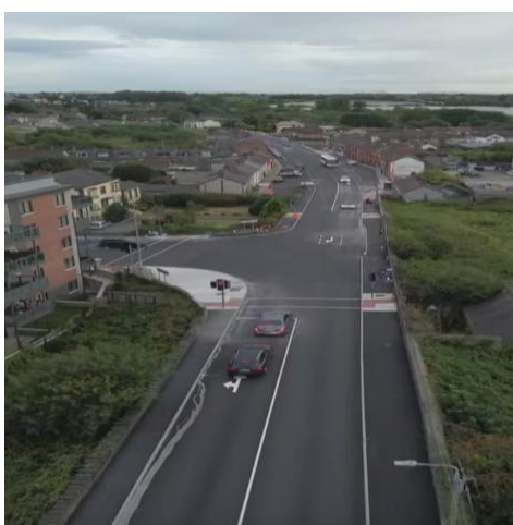
Hill Street Bridge
