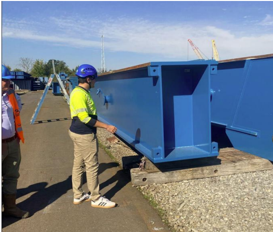
Temporary Skid track Beams
