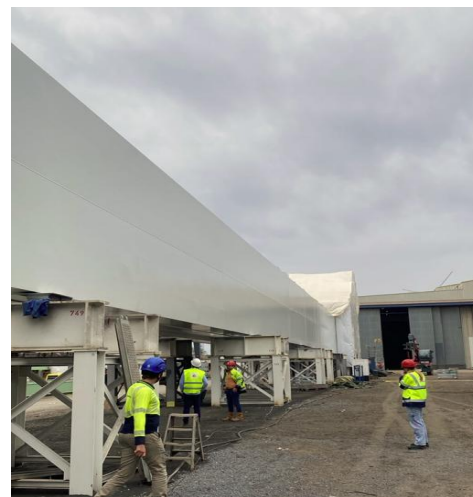
Completed Pylon Section.
