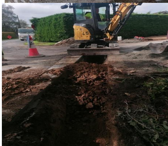
Figure 4 – Drainage Works on L-6300, Hill of Rath
