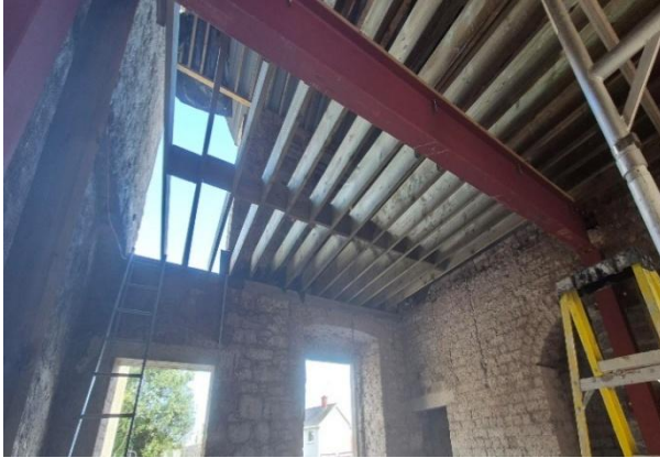
Judges Chamber roof repair
