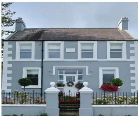
Restoration of Oberon Villa, Omeath
