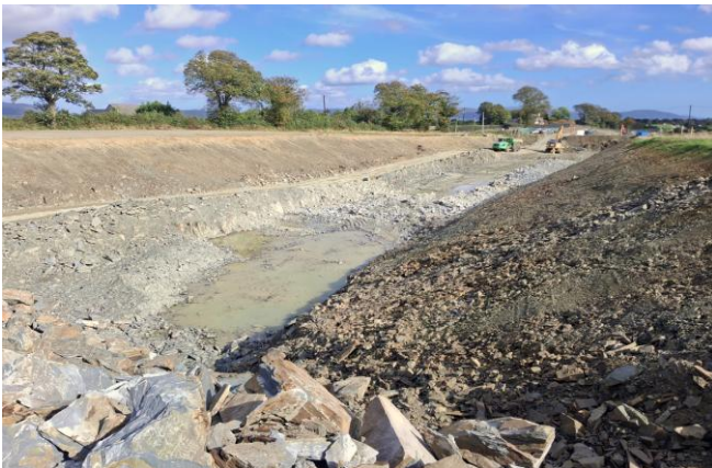
Earthworks cutting on the N53
