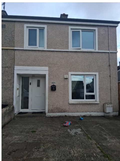
EERP works completed at property in Doolargy, Dundalk which included windows, doors, attic and heat pump
