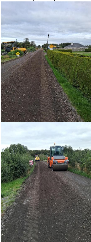
Figure 1 – Resurfacing on L-5232, Townparks
