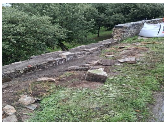
Figure 5 - Repair to Stone Wall at Woodmill, Tullyallen after RTA
