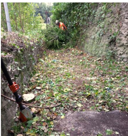
Vegetation removal to the rear of West gate House
