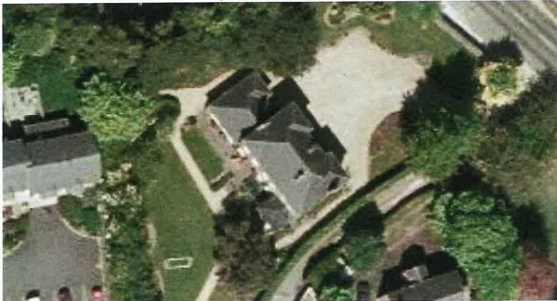
Above: Aerial image of subject dwelling taken 2 nd May 2007 showing conservatory and no extension.
