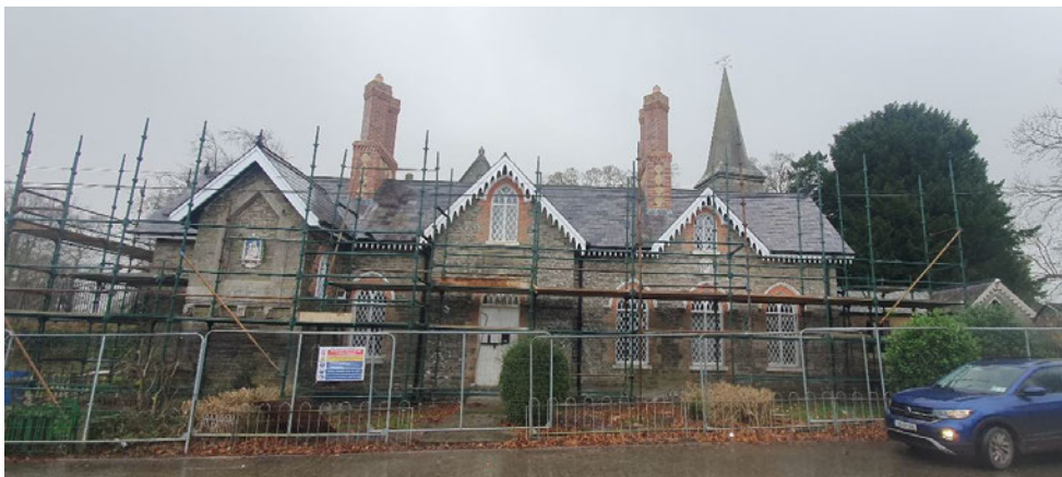
Conservation works so far, showing new chimneys
