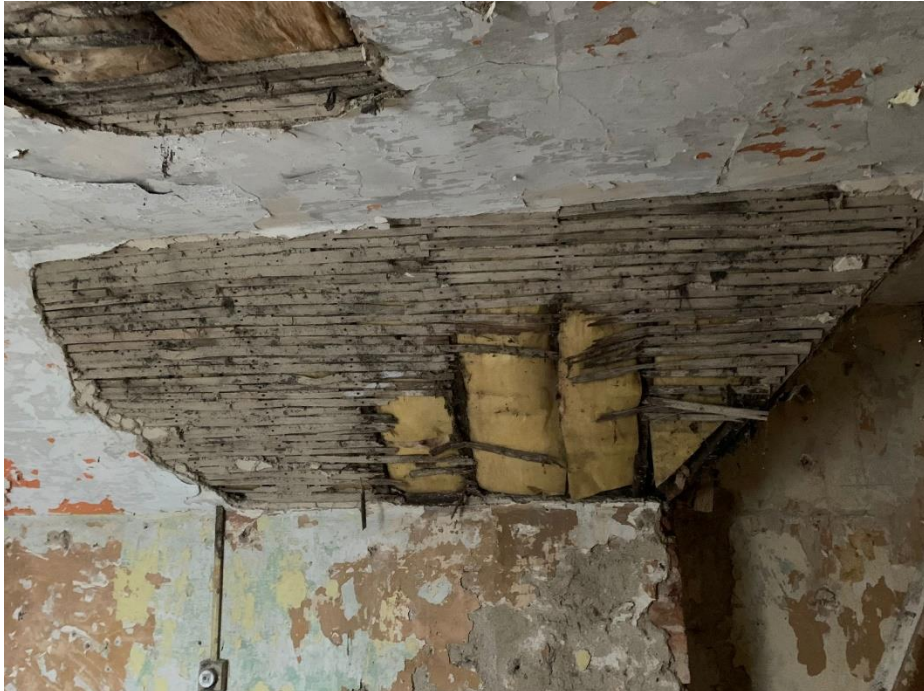
Damaged lathe and plaster ceilings
