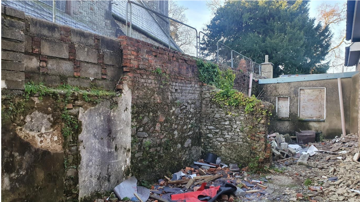
Photo showing blockwork section of retaining wall
