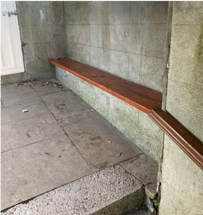
Additional support required to bench
