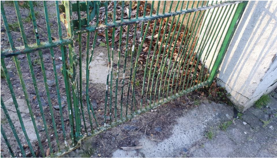
Deformed steelwork
