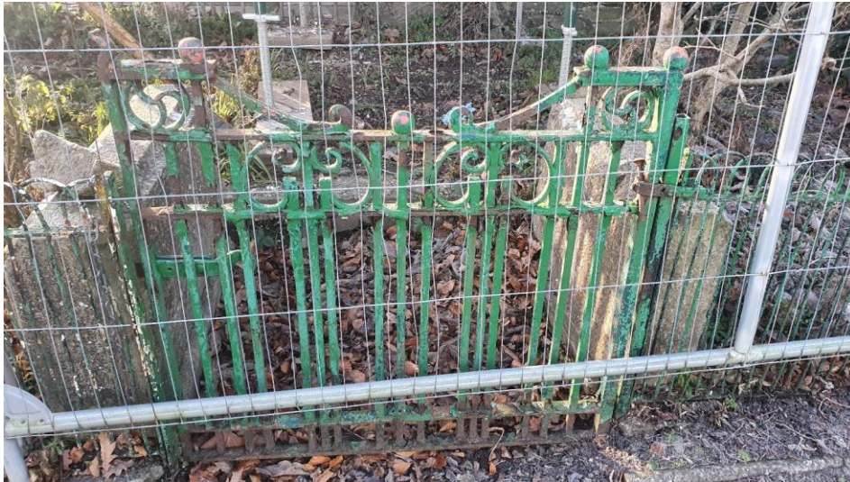
Small iron pedestrian gate
