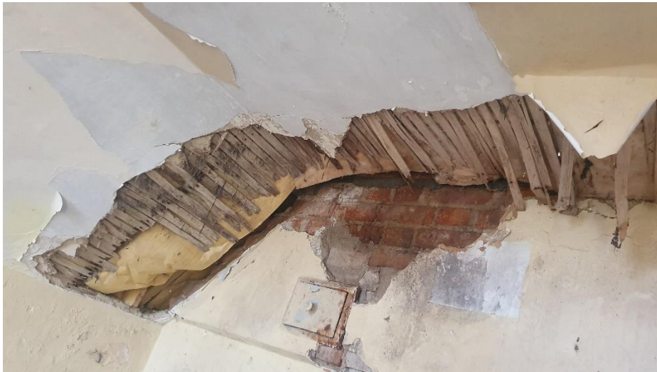
Damaged lathe and plaster ceilings
