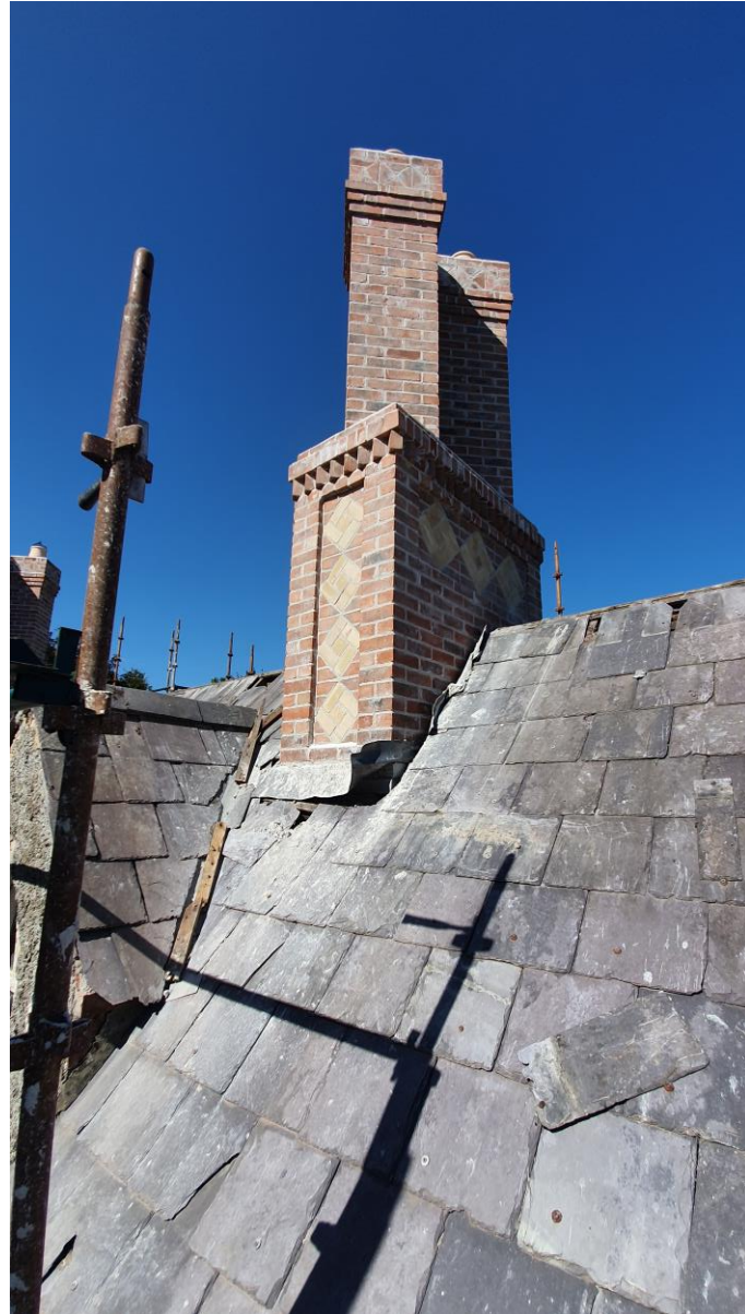
Chimney restoration as part of HSF grant 2023.
