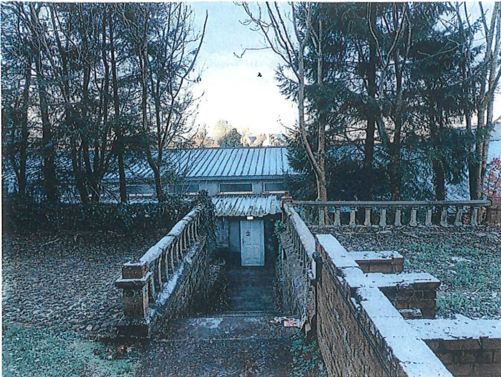
Figure 3: Views of existing swimming pool building roof.
