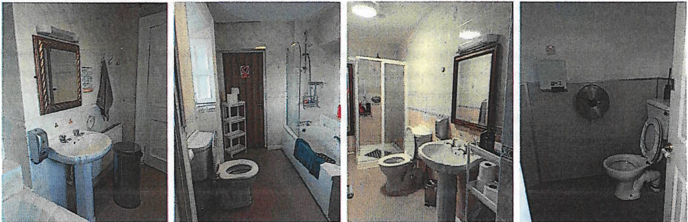
Figure 1: Views of some of the existing bathrooms to be replaced (all internal works).
