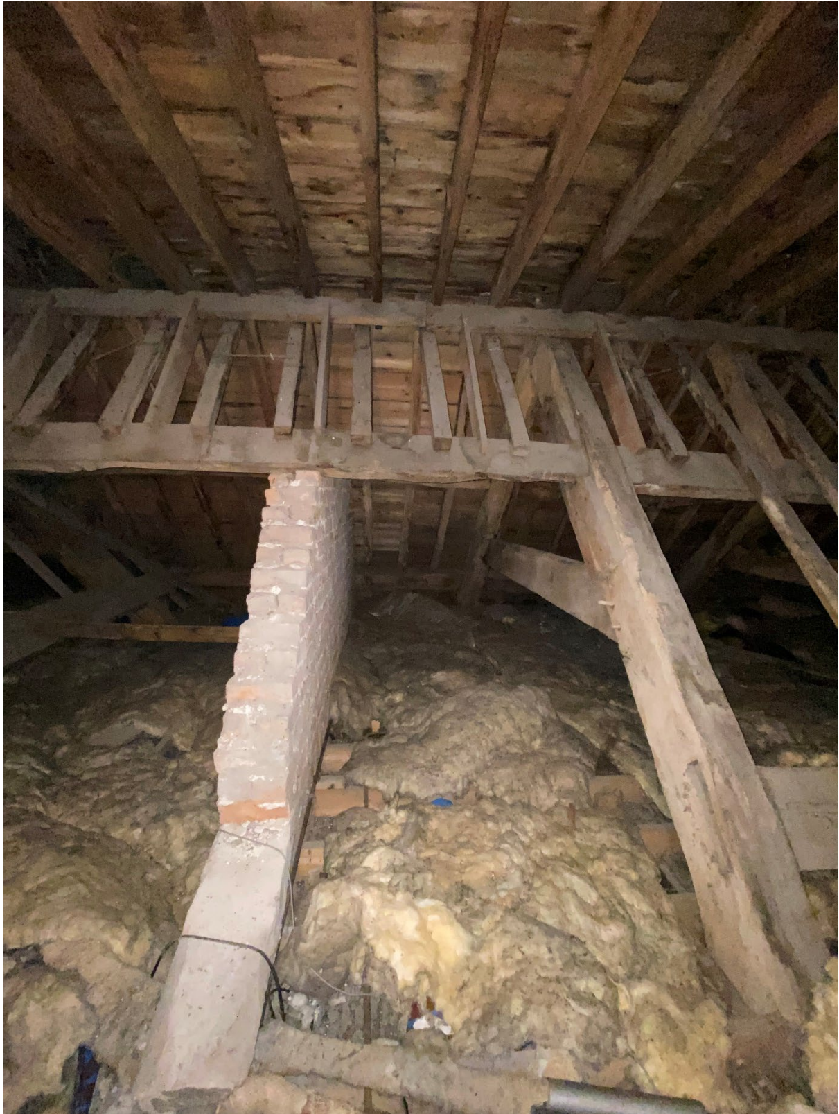
S57 – Beaulieu House (Roof Timbers)
