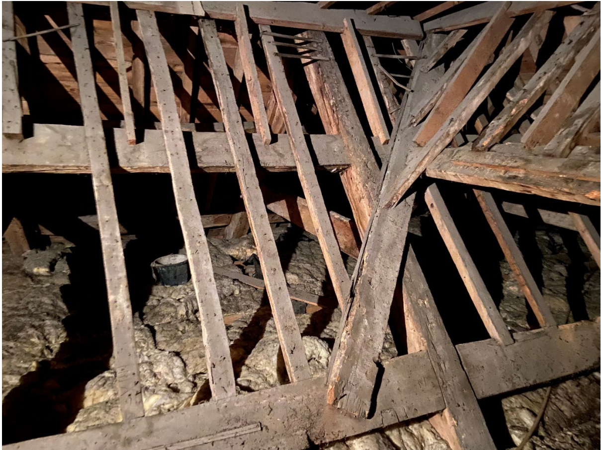
S57 – Beaulieu House (Roof Timbers)
