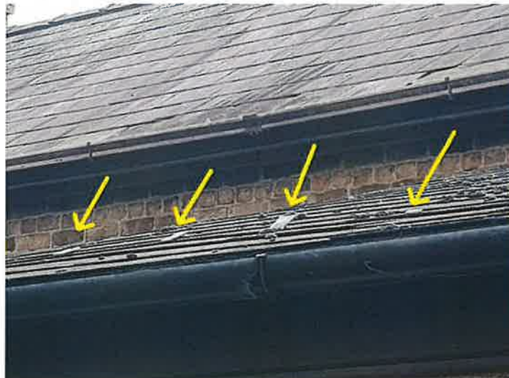
Metal / lead clips supporting roof slates to roof.
