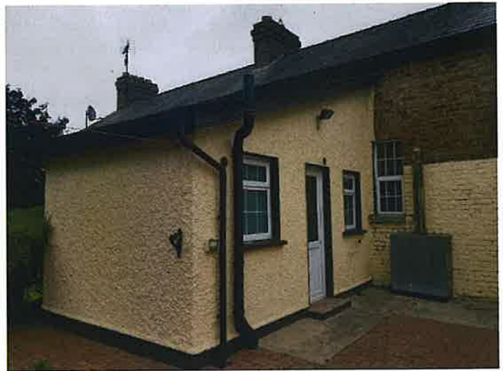
Rear extension added.
