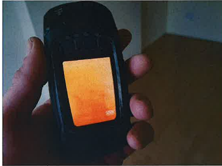
Ceiling dry at time of inspection.
