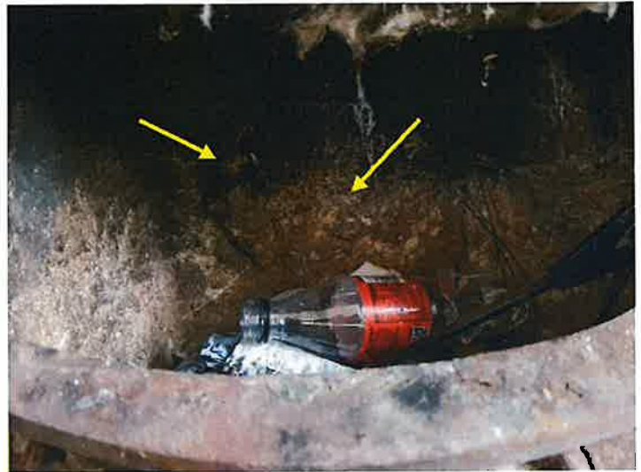
Repair/ replace damaged firebrick in fireplace.
