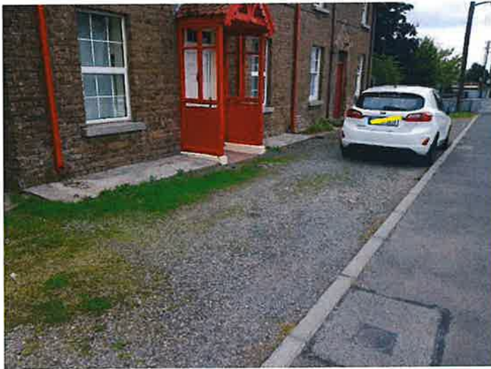
Front of property.
