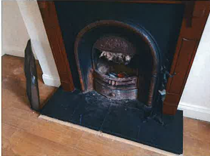
Chimneys providing ventilation to rooms.
