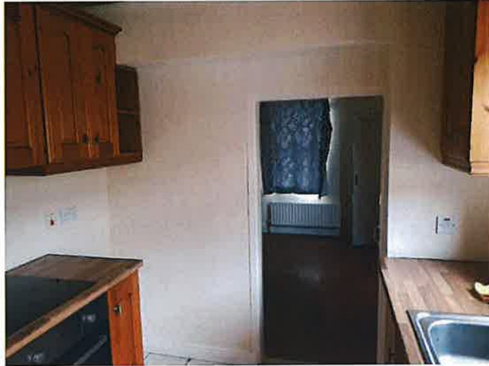
Wall removed / widened between original house and rear extension.
