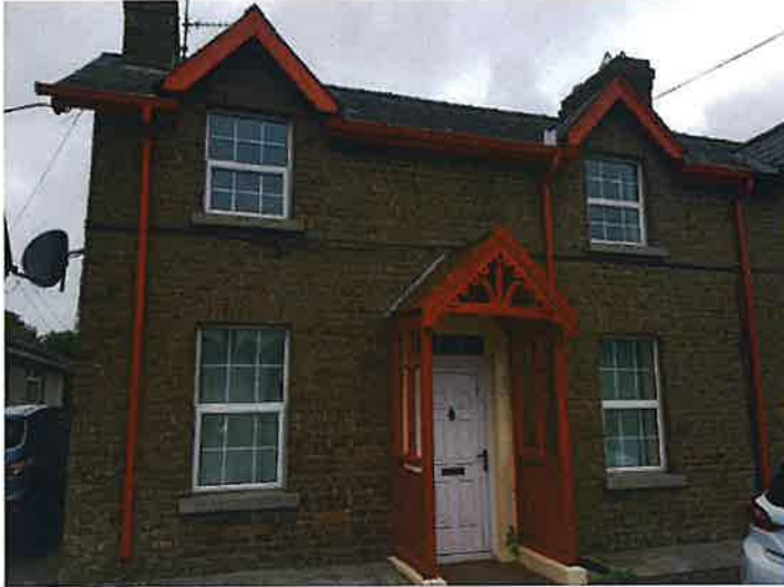
Front of property.
