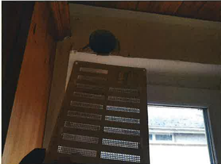
Re-fit cover to kitchen vent
