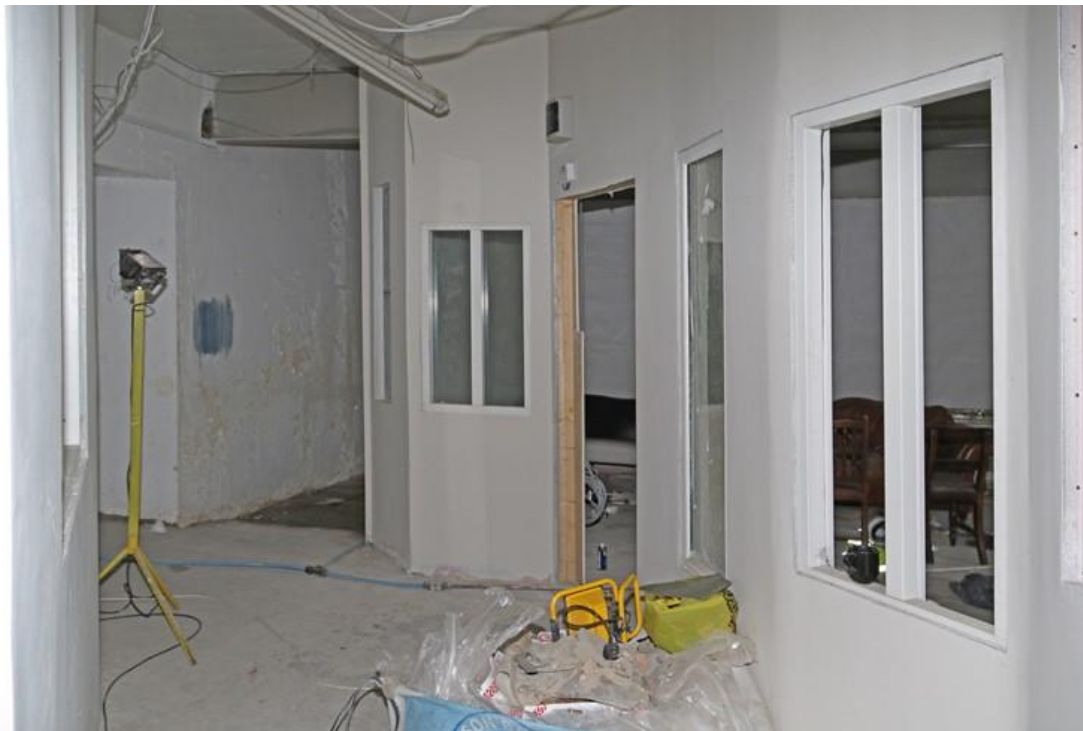
Plate 19: GF-4: Passageway through ground floor room GF-4
