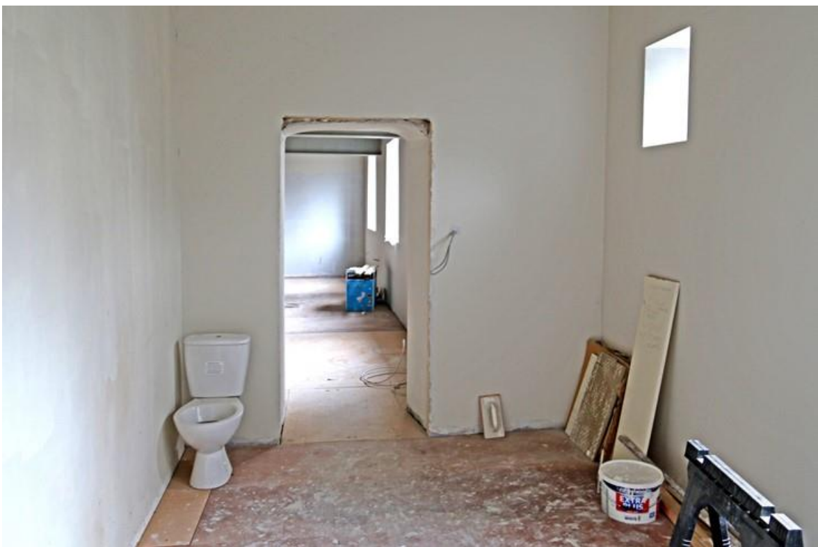
Plate 33: FF-4: WCs at rear of return
