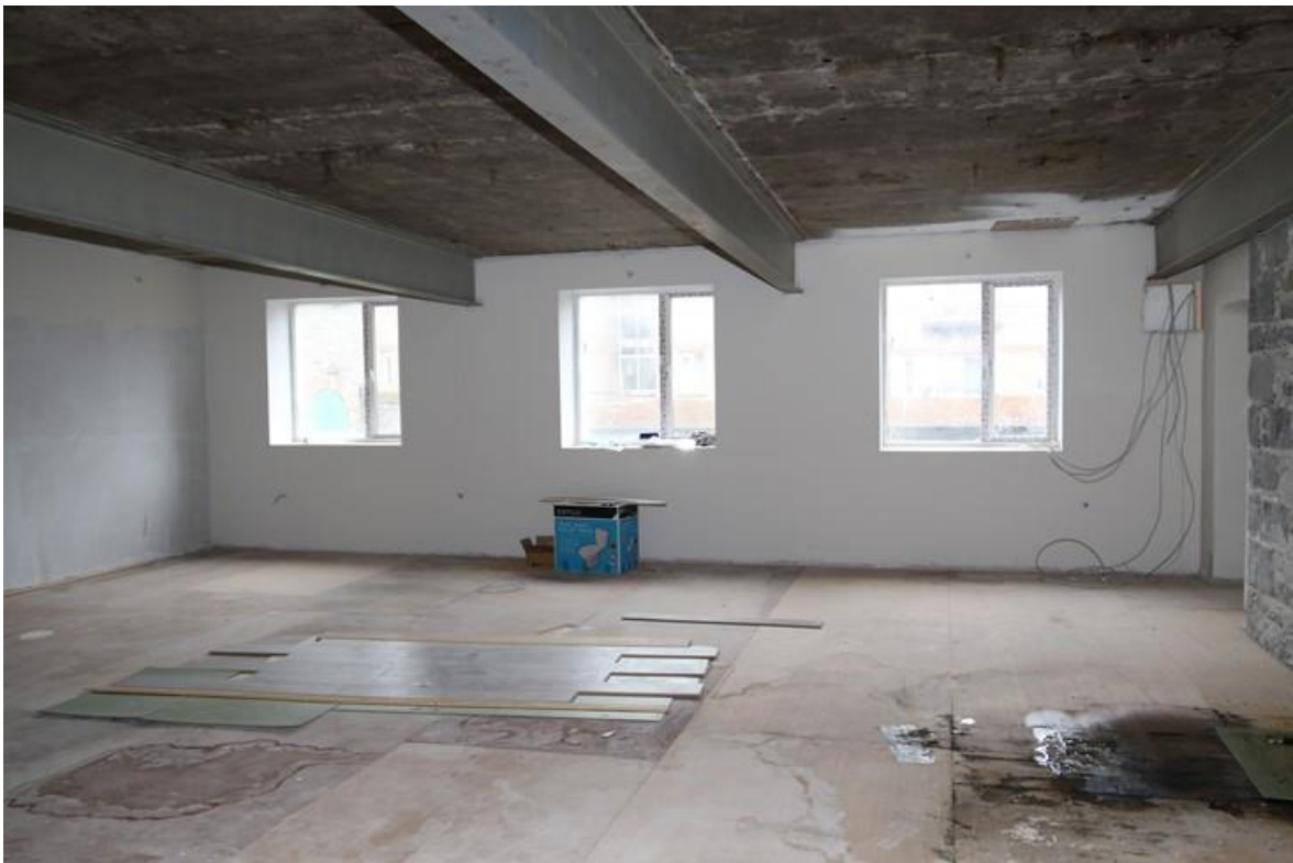
Plate 28: FF-3: First-floor rear room in extension
