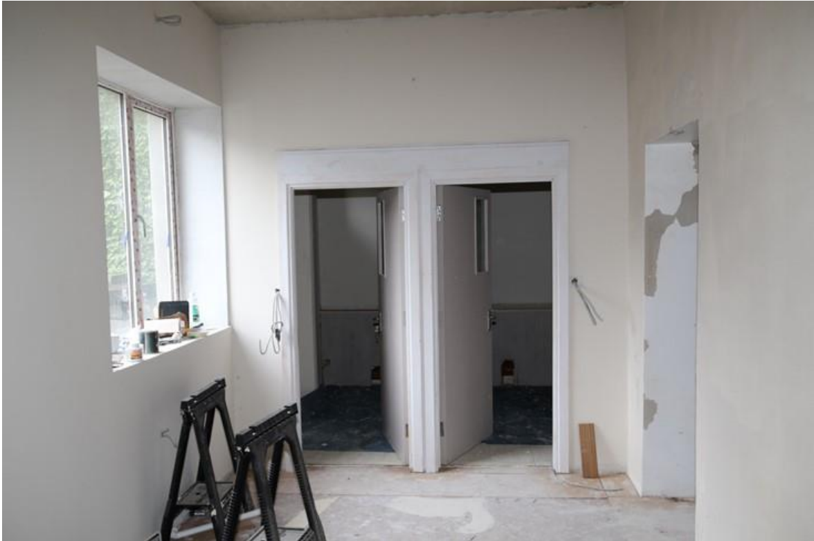
Plate 32: FF-4: WCs at rear of return
