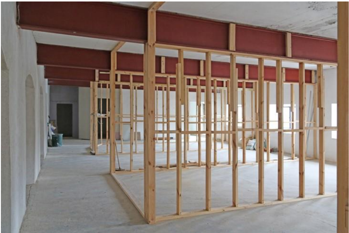
Plate 27: FF-2: Eastern end of first-floor main room
