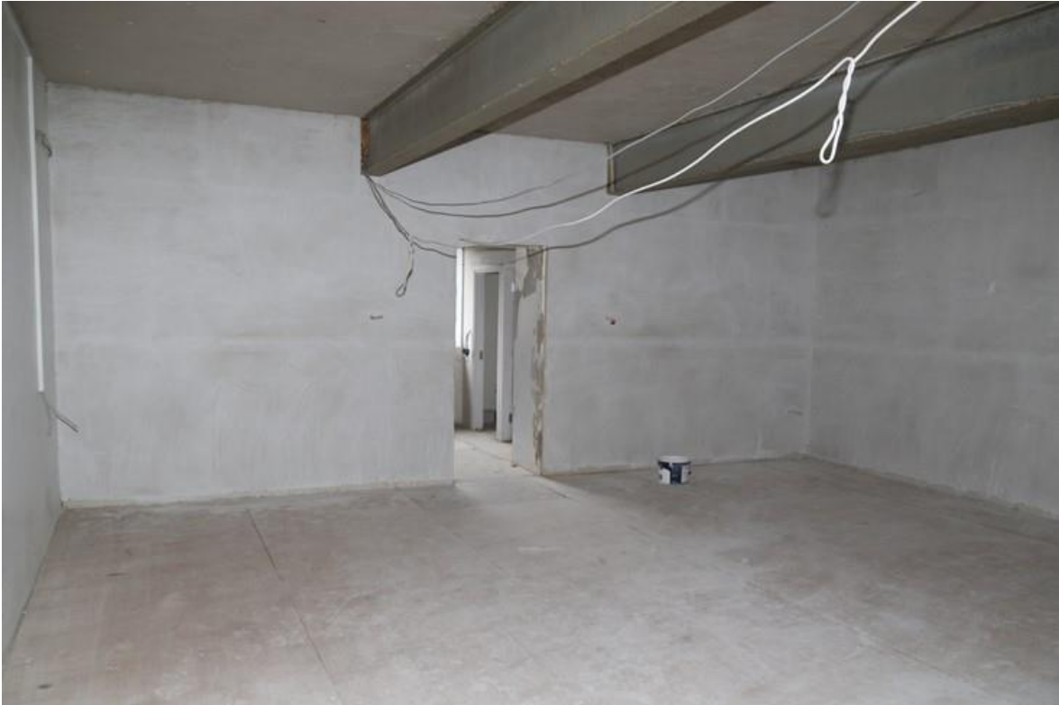
Plate 30: Room FF-4: Eastern return at first floor
