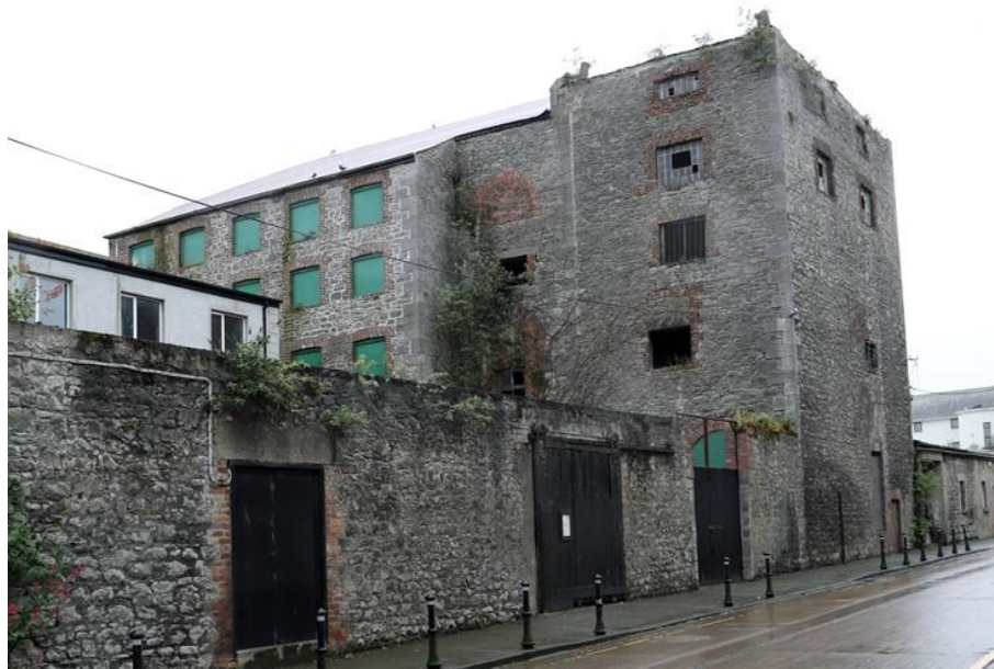
Plate 6: Rear return, viewed from north-east
