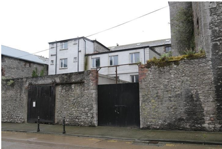
Plate 8: Gateway and rear boundary to North Strand
