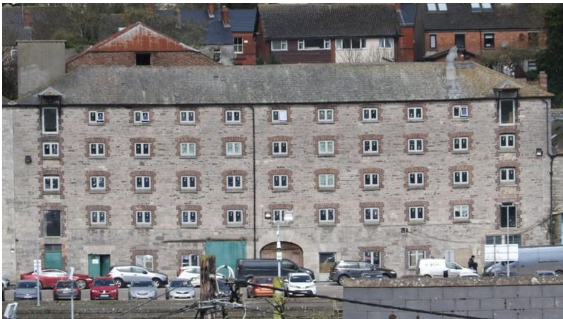
Plate 44: Frontage of building
