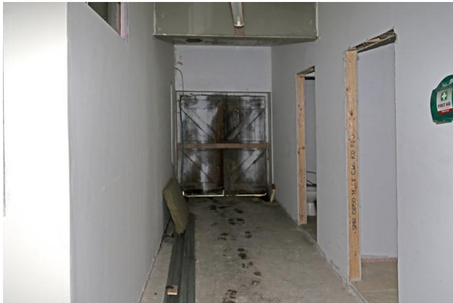
Plate 23: GF-6: Extension to north of main building with doors to yard
