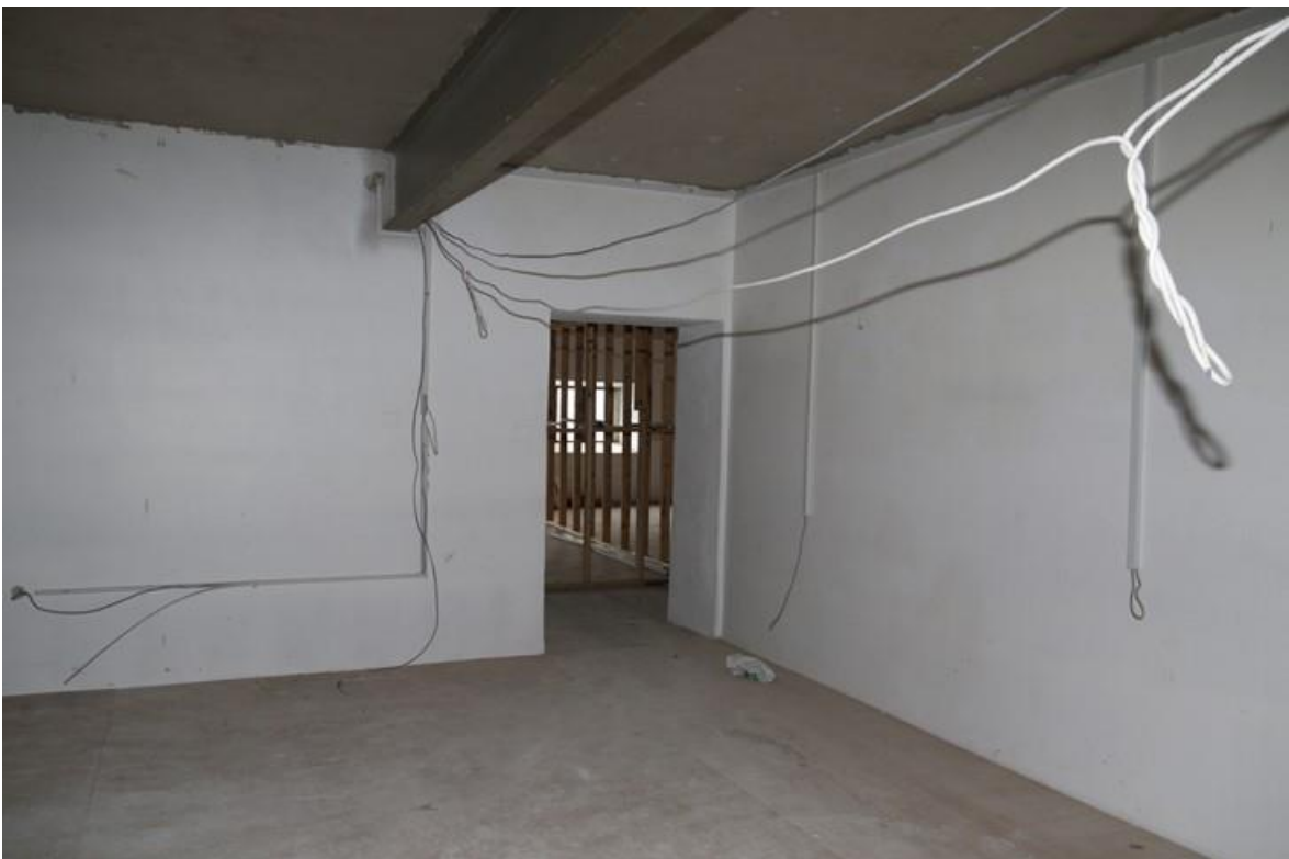
Plate 31: FF-4: Main room in rear return, looking towards main building
