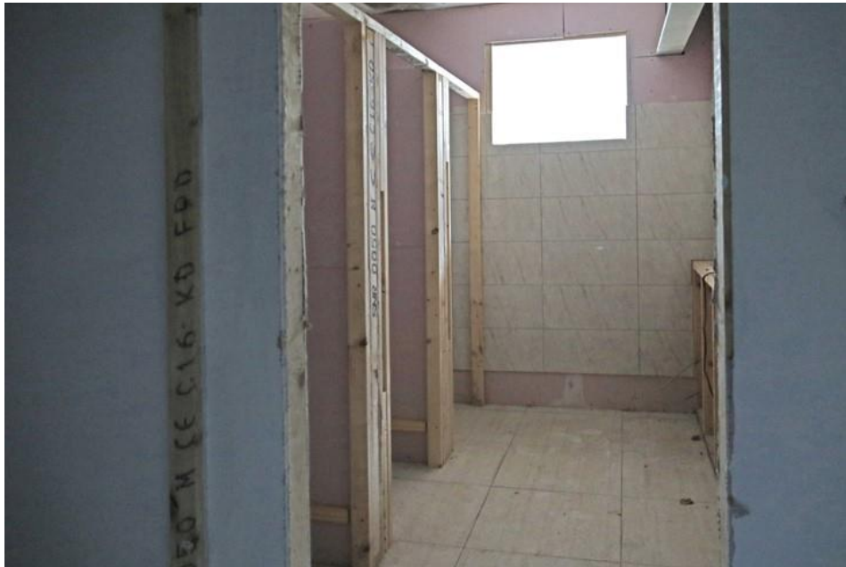
Plate 24: GF-6: WCs in extension to north of main building
