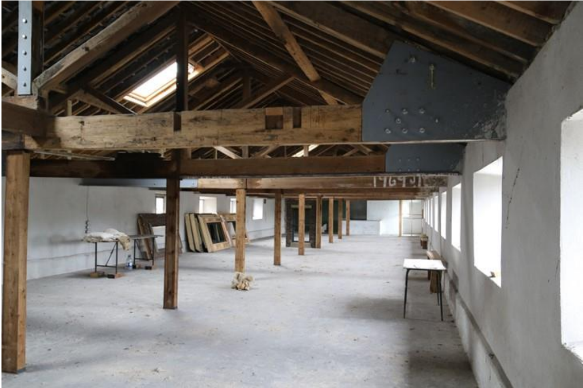
Plate 39: TF-1: Third-floor main room
