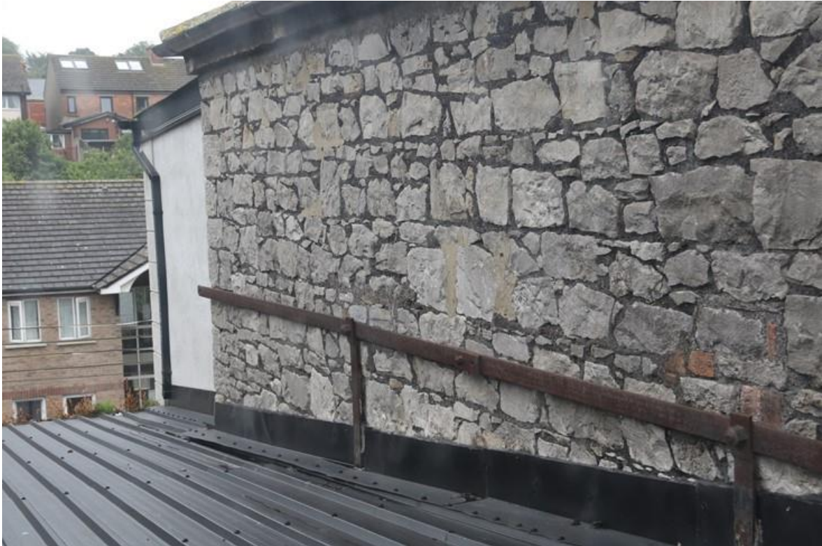
Plate 45: Top of original eastern return, seen from main building
