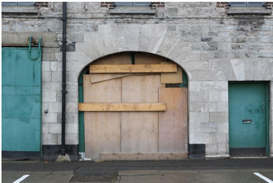
Plate 10: Carriage opening and doorway, front elevation
