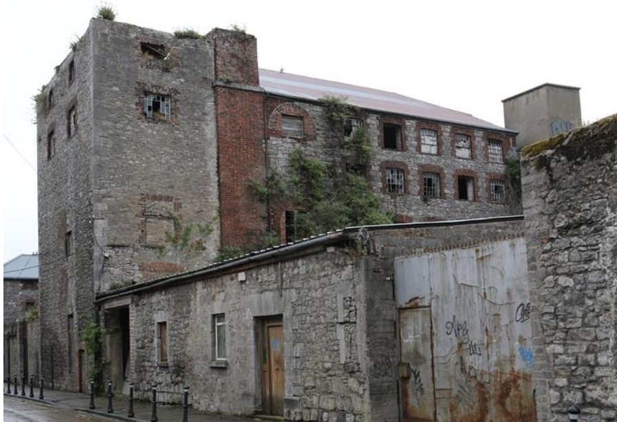
Plate 4: Mill and engine house as seen from North Strand, to west
