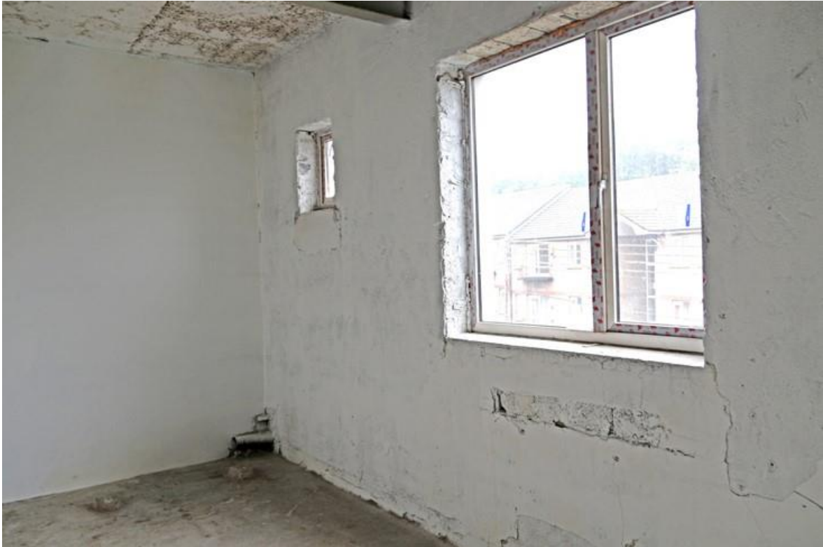
Plate 37: SF-3: Former toilets at rear of return
