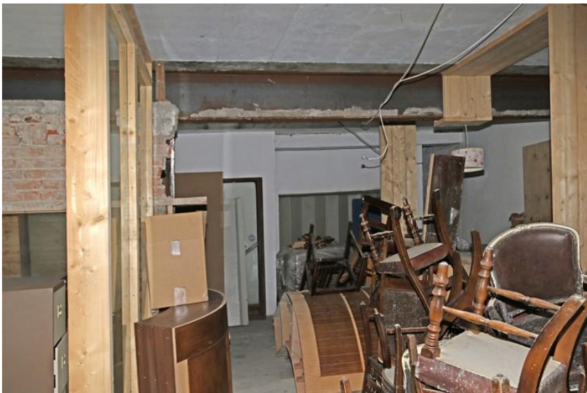
Plate 14: GF-1: Ground floor room 1, lift
