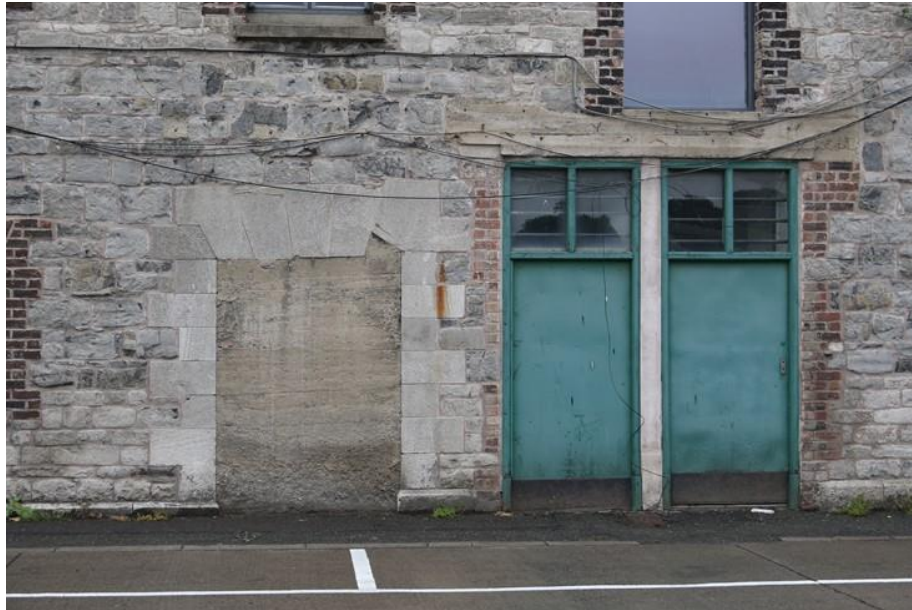
Plate 11: Door openings, front elevation east
