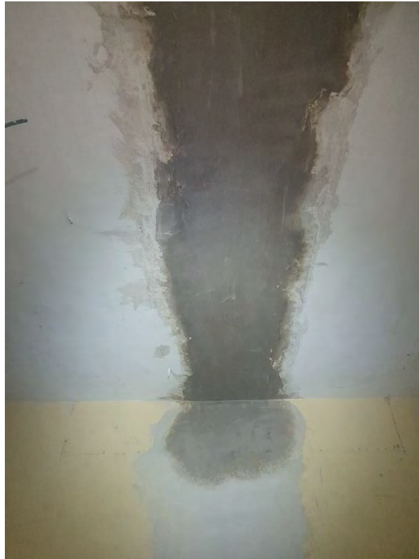
Image 3 – View of repaired ceiling plasterwork (unpainted).
