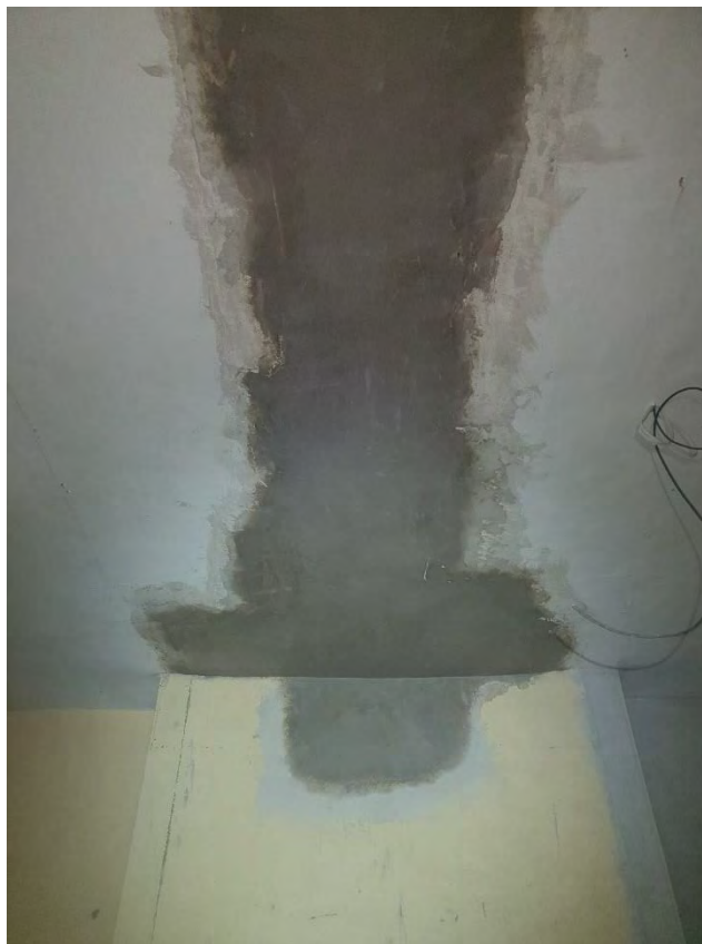
Image 4 – View of repaired ceiling plasterwork (unpainted).
