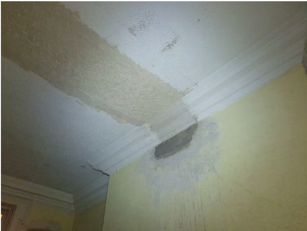
Image 6 – View of repaired ceiling plasterwork (unpainted) and cornice details.
