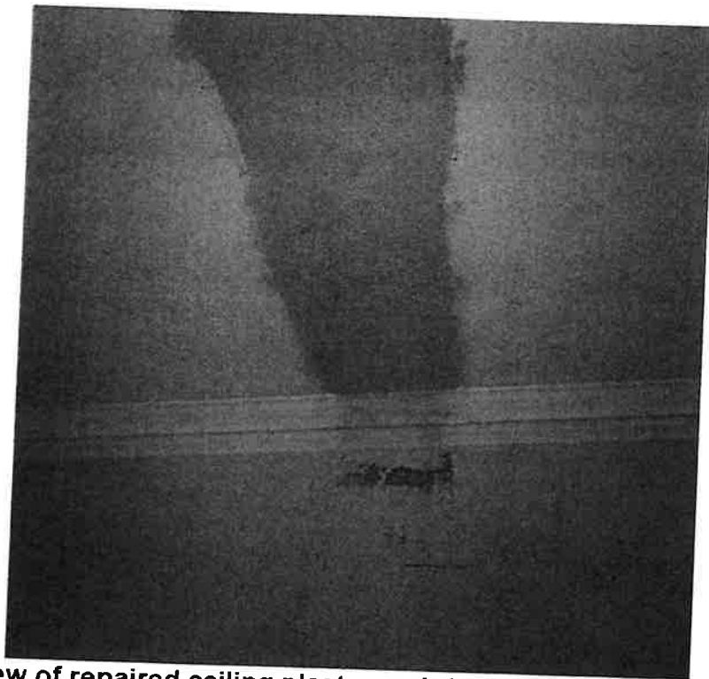
Image 4 – View of repaired ceiling plasterwork (unpainted).
