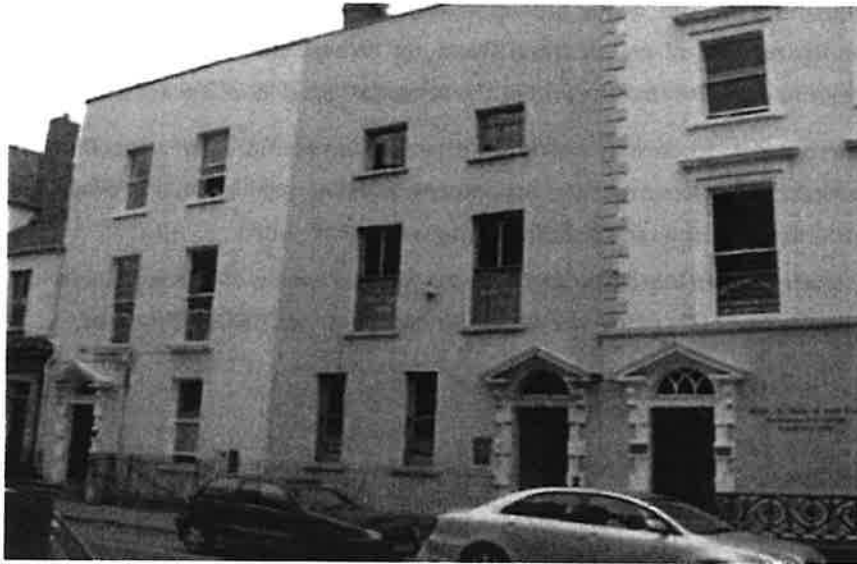
Figure 1: Front Façade – 29 St. Laurence Street, Drogheda
