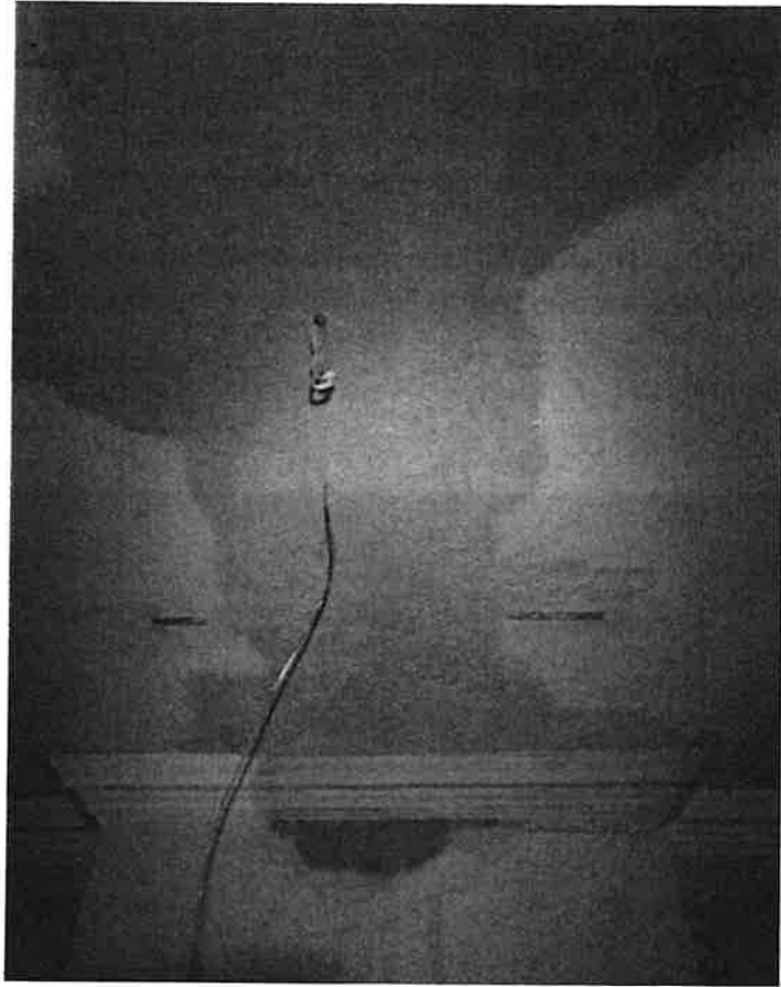
Image 2 – View of repaired ceiling plasterwork (unpainted) and cornice details.
