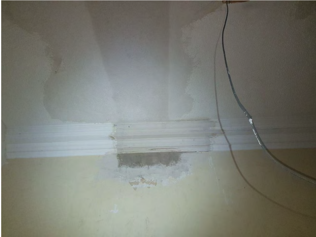
Image 1 – View of repaired ceiling plasterwork (unpainted) and cornice details.
