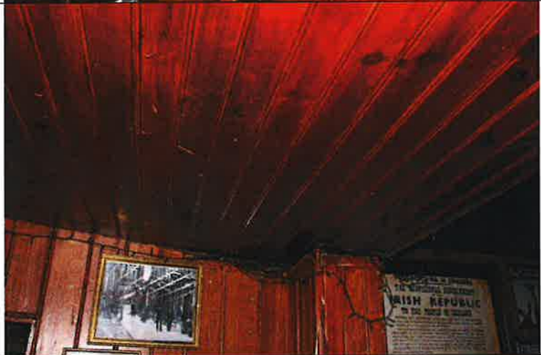
Tongued, grooved and rounded boarding of ceiling. (3947)
