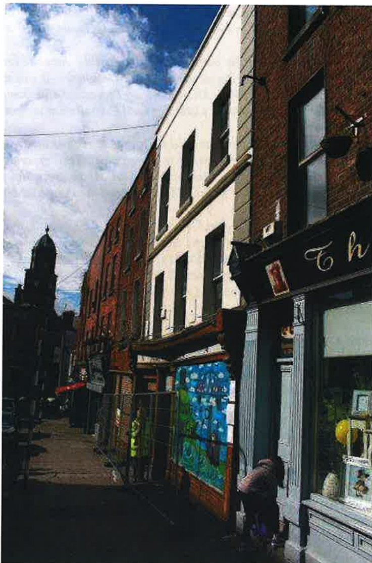
Figure 6: Peter Mathew's Pub with its rendered front and fascia with a large deflection.
