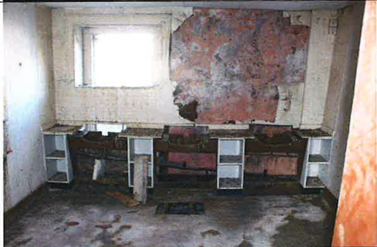
Second floor front room (5236)
