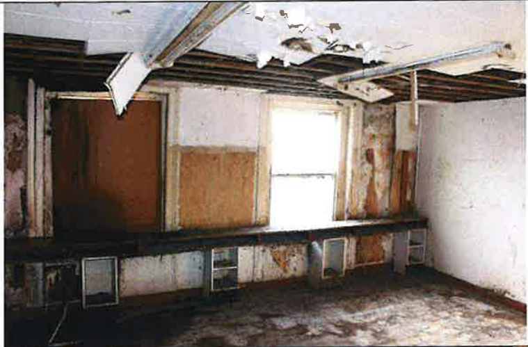
Second floor front room (5234)
