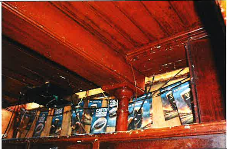
Detail of beam surround and cast-iron column. (3939)
