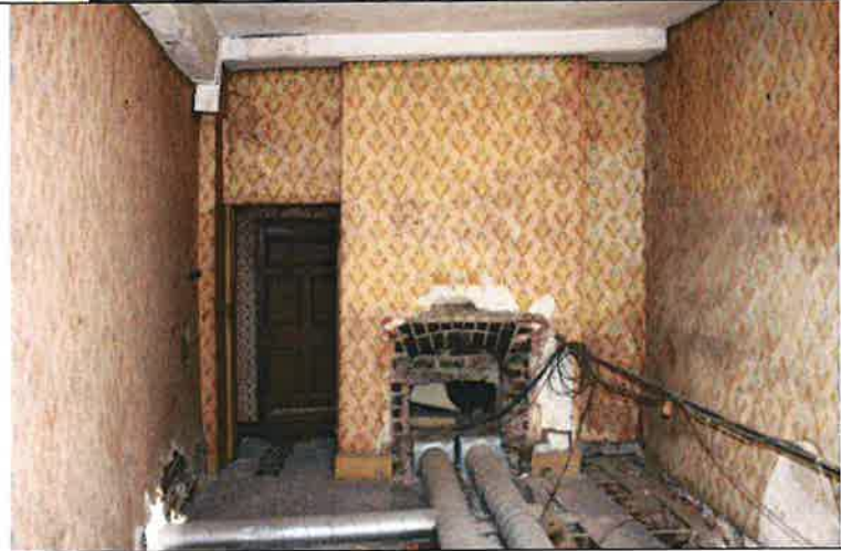
Smaller room on the first floor. (3764)
