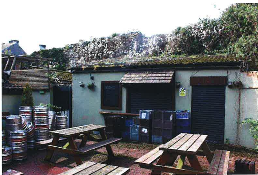
Figure 12: Modern stores at rear of no. 8. (3738)
