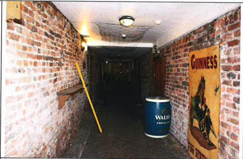
Entrance corridor, the plaster has been removed. (3745)
