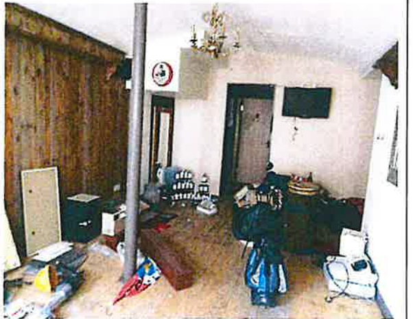
FIGURE 12 GROUND FLOOR SPINE WALL REPLACED BY COLUMN
