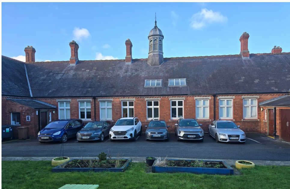
Image of roof where 14 solar panels to be erected.
