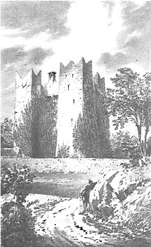
View from the South West (unattributed) shows the castle front with machicolation and chimney stack above the main entrance. The main entrance area is shown overgrown with creeper suggesting that it was disused at this time. There appears to be a steep escarpment in front of the castle.
