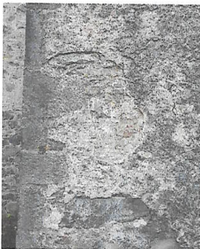
Earlier lime render over-rendered with Portland cement material.
