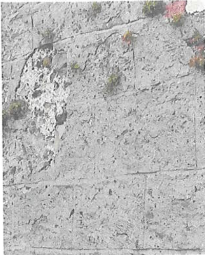
Cement render over lime render. Incised lines in render.
