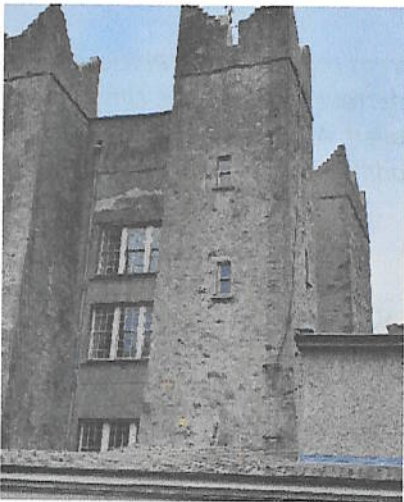
Rear façade showing rendered blockwork infill at window insertions and older render on turret.
