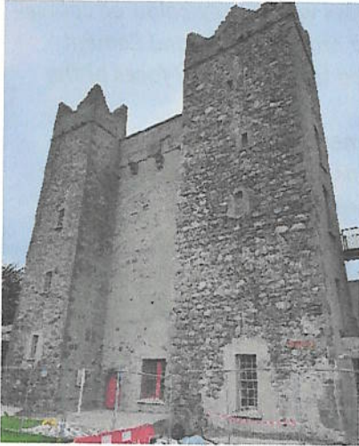
Entrance faced showing cement render to the centre, side of turret and around windows.
