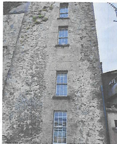
Rear façade showing rendered blockwork infill at window insertions and older render on turret.
