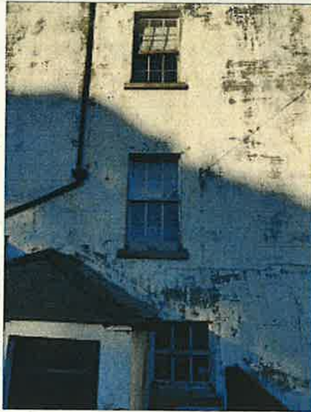
Photograph 1- 3no. windows on the south facing elevation (rear of house)
