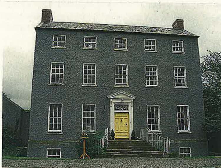
Figure 1 - Front (North) facade
