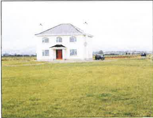
No shelter on an exposed coastal site
