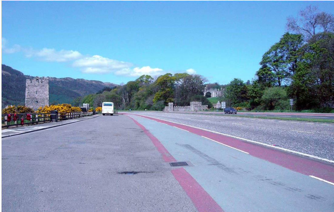
Plate 3.2 Existing parking adjacent to Narrow Water Keep
