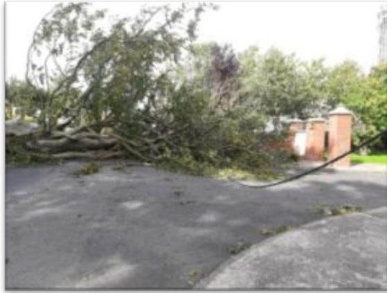
Figure 3.4 Fallen tree and damaged overhead wiring due to fallen tree in Omeath
