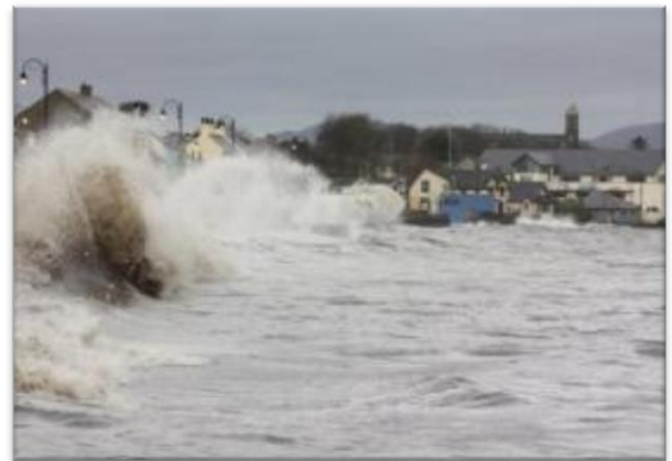
Figure 3.3 Flooding in Blackrock Main Street due to storm surges in 2015.
