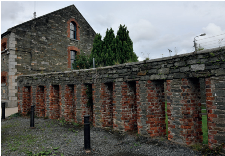
Exercise yard wall today with former 'A' wing cell-block behind.
