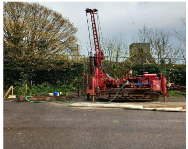
Bore Hole Rig
