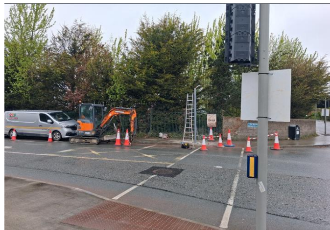
Figure: traffic light repairs
