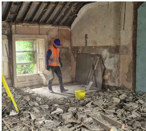
Clearance of debris within Judges Chambers
