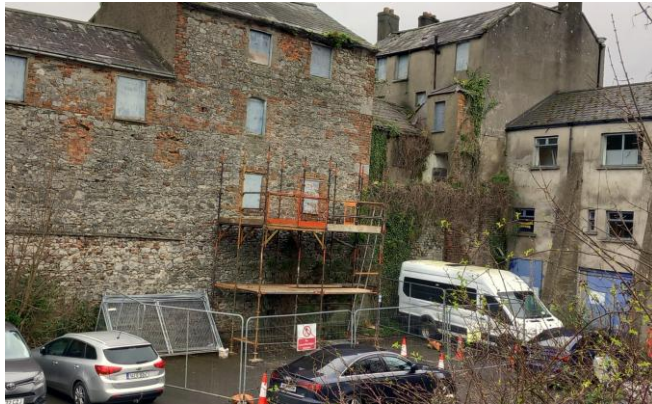
Scaffolding erected for access as part of Safeguarding Works
