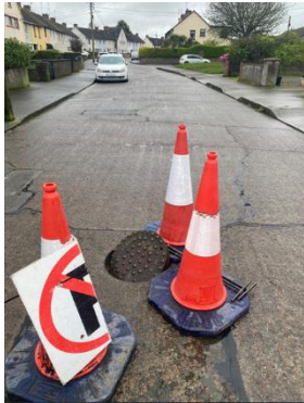
Figure: Manhole Repair
