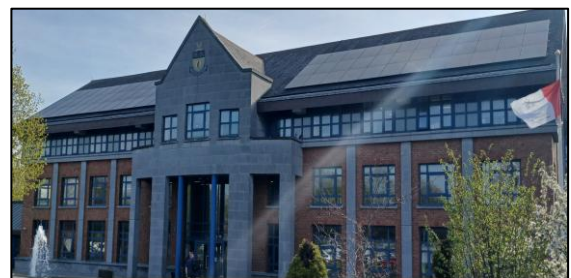
New Solar PV at County Hall Dundalk
