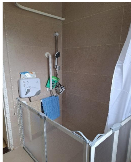
Bathroom Adaptation completed in Drogheda with funding provided with a HAG
