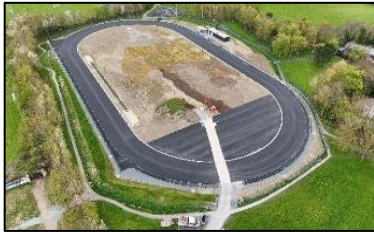
The New Dundalk Athletics Track (under construction)
