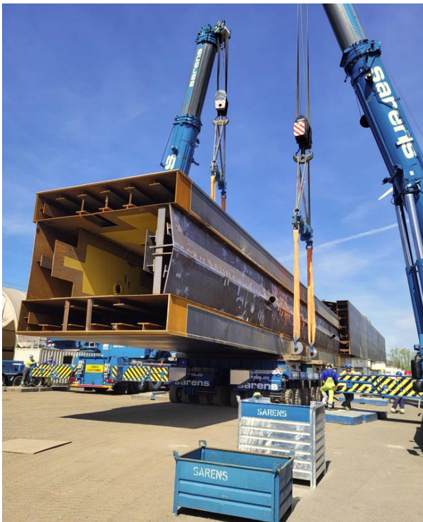
Section 2 of Pylon moved into yard for welding to section 3.
