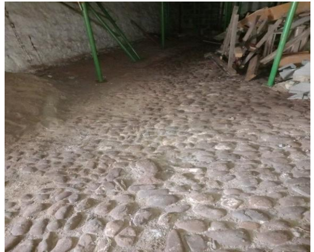
Internal cobble floor within West Gate House
