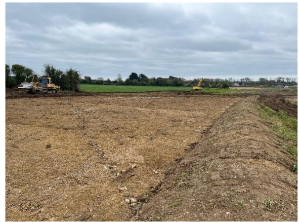
Topsoil stripping at Main Line north of Aston Village
