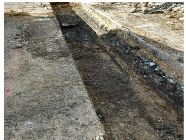
Slit Trench Excavation
