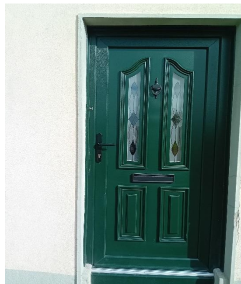
New front door completed in Tallanstown, with funding provided with a HOP
