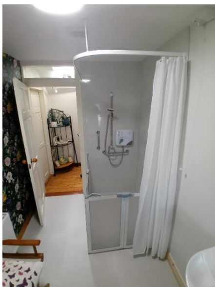
Bathroom Adaptation completed in Dundalk with funding provided with a HAG
