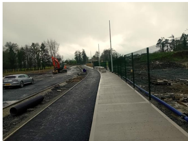
External footpath works under construction
