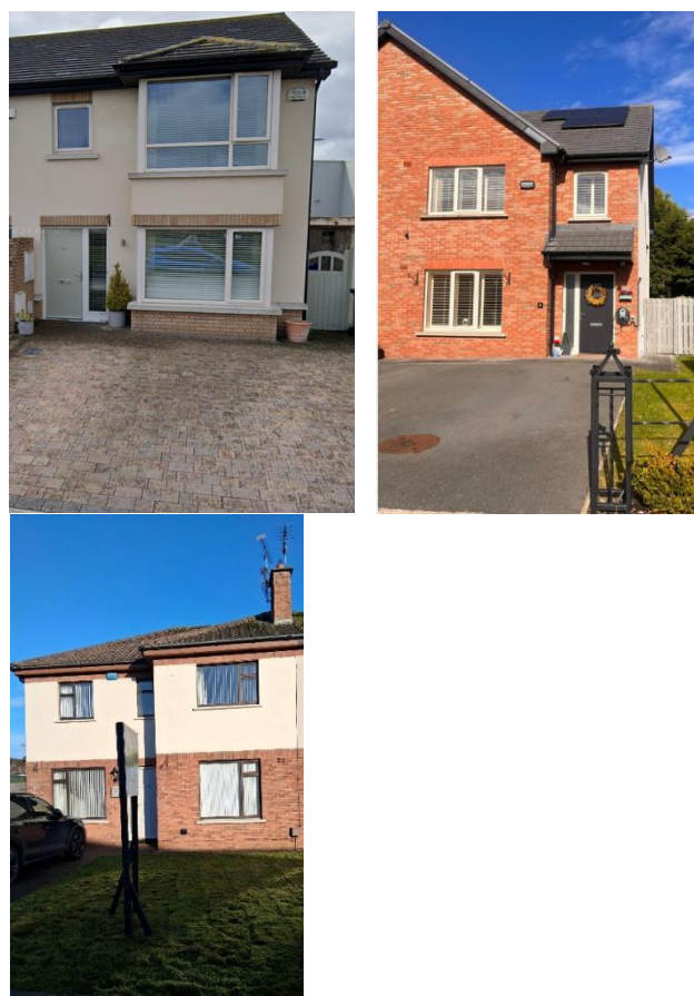
Recently acquired properties in Blackrock and Dundalk
