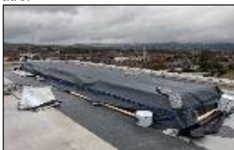
Photos: Roof vents under construction at Dundalk Town Hall
