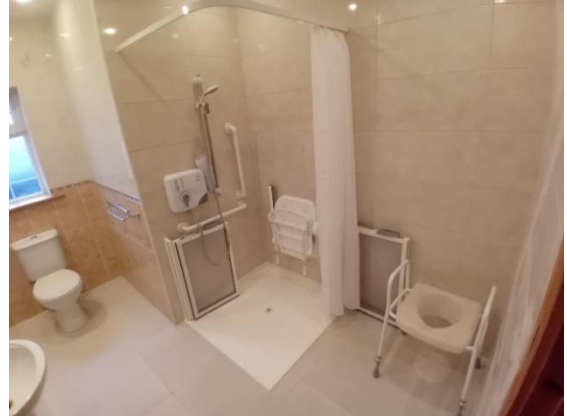
Bathroom Adaptation completed in Drogheda with funding provided with a HAG
