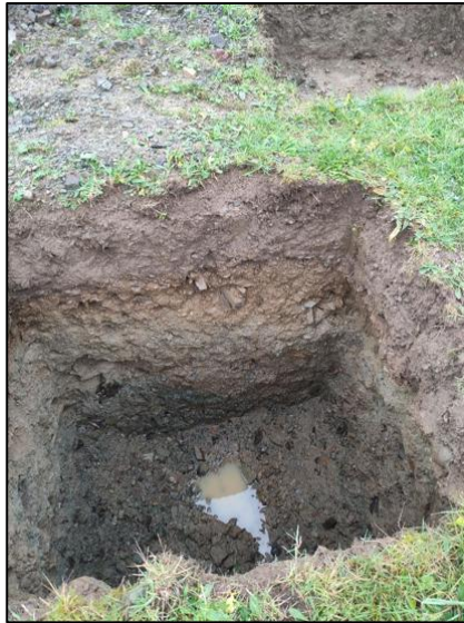
Trial Hole Inspection
