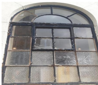
Carlingford Library window before conservation works
