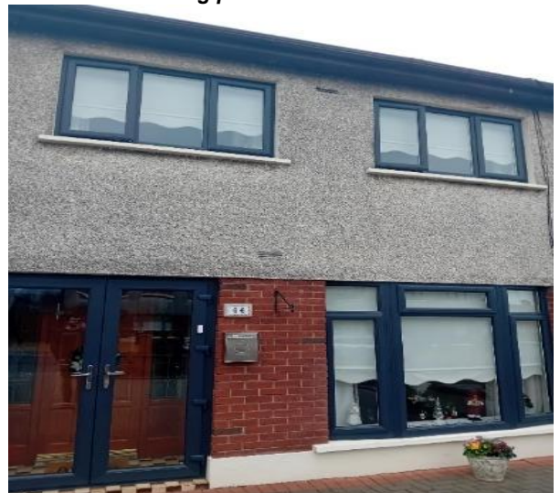
New Windows and Door completed in Drogheda, with funding provided with a HOP
