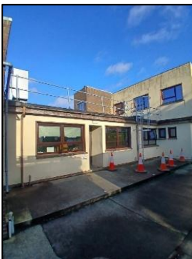
Photos: New access and egress at roof of Dundalk Fire Station
