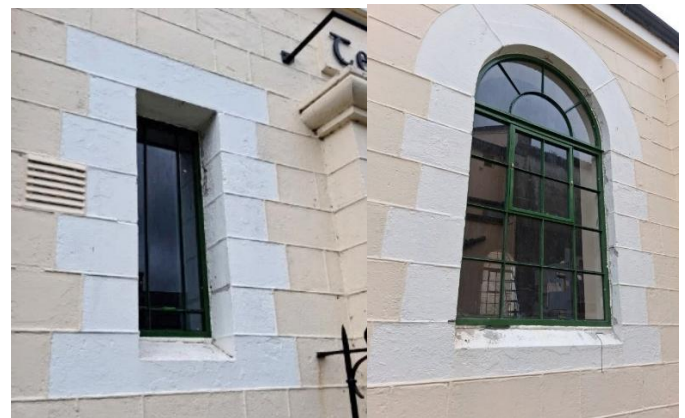
Carlingford Library windows after conservation
