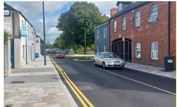
New road surfacing on Linen Hall Street.
