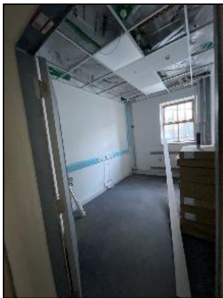
Photos: Refurbishment Works at Cornmarket Building, Fair St, Drogheda
