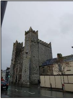
Photos: Upgrading Festive Lighting at Ardee Castle
