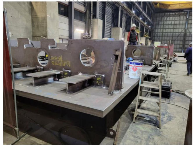
Fabrication of back plate for fixed span pylon.
