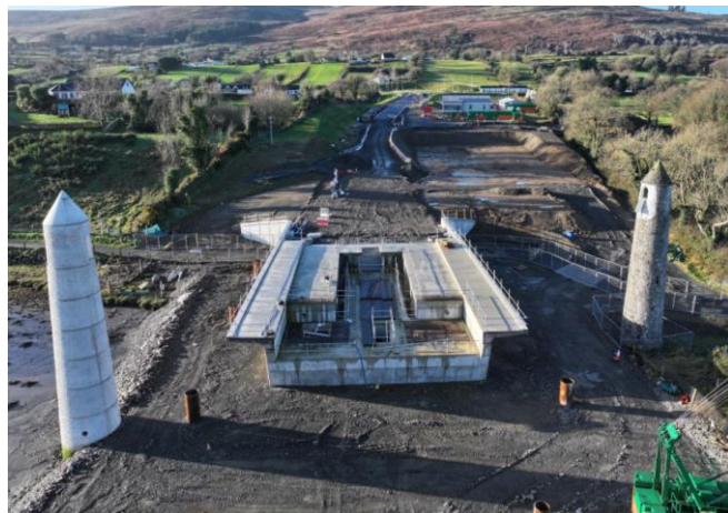
Temporary works for Crawler Crane platform ongoing, southern embankment.
