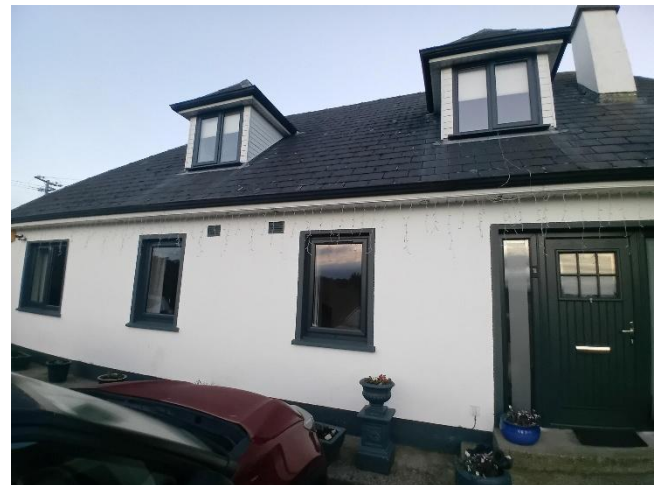
New Windows and Door completed in Drogheda, with funding provided with a HOP
