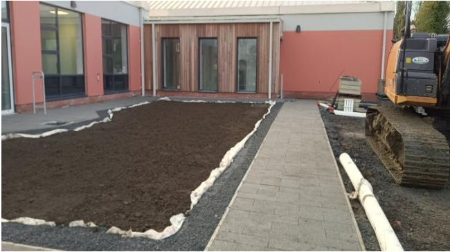
External works under construction (11/12/2025)
