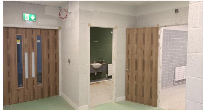
Internal school finishes (11/12/2025)
