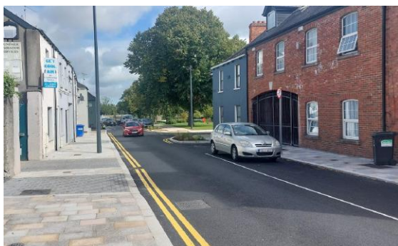
New road surfacing on Linen Hall Street.
