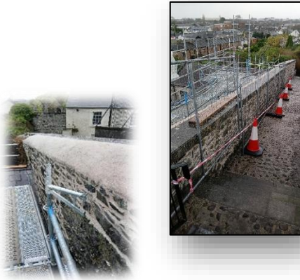
Photos: Completed Wall conservation works at Millmount
