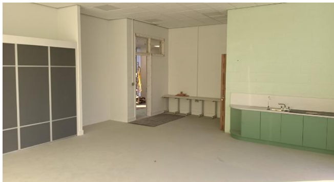
Internal school finishes (11/12/2025)
