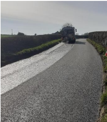
New Surface laid on L-2310, Ballymakenny
