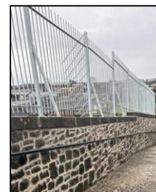
Wall stabilisation and new railings at Millmount
