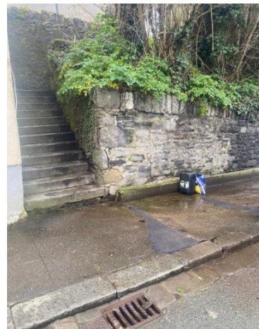
South Louth Roads Area clean and jet gully on Marys St – to prevent surface water flowing onto road
