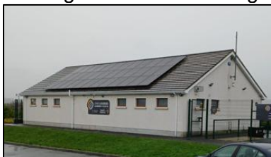
Solar PV is complete at the Lourdes Stadium
