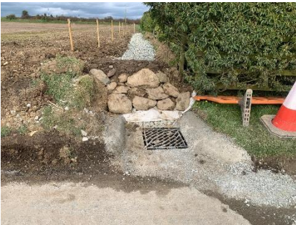
Drainage Works on L-6304, Milltown Lane
