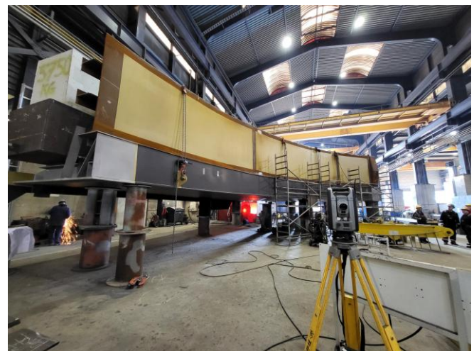
Section of Pylon Boot in assembly.
