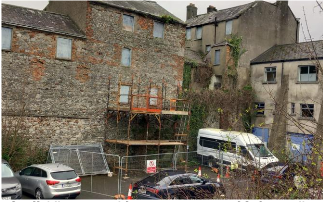
Scaffolding erected for access as part of Safeguarding Works
