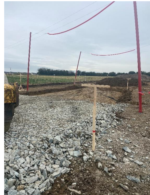
Topsoil stripping of the mainline, near Sandpit Rd.
