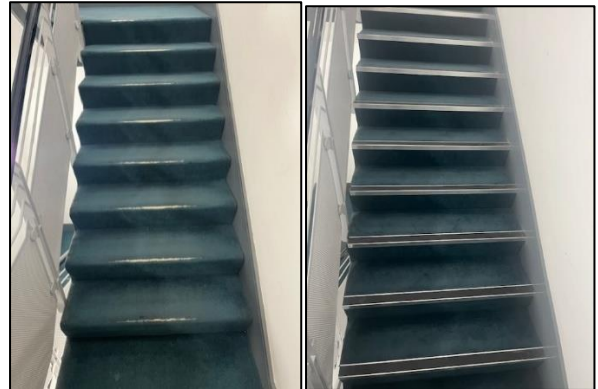
Image shows stairwell before & after Works
