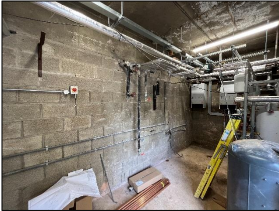
Dundalk Fire Station's Plantroom Progress
