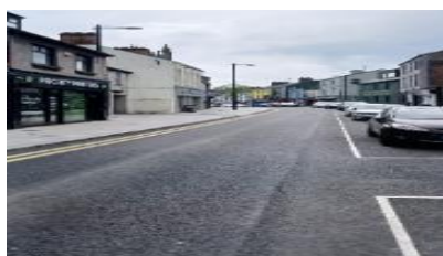
Bridge Street (Phase A) – Overhead cables and ESB Poles removed
