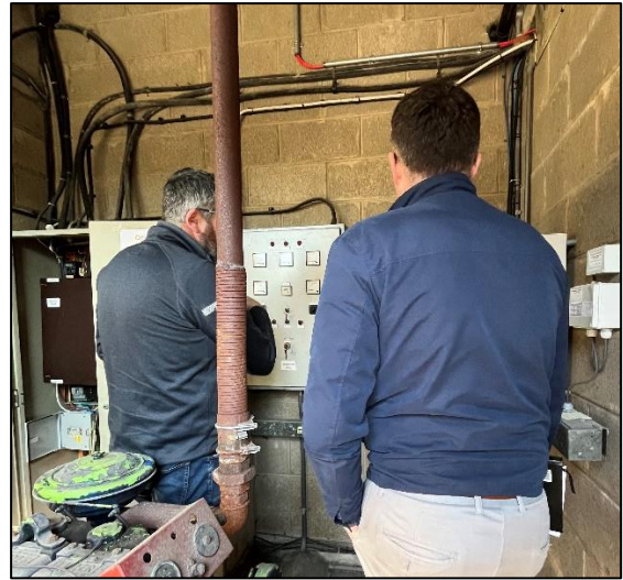
Meeting going over the Electrical Infrastructure Works
