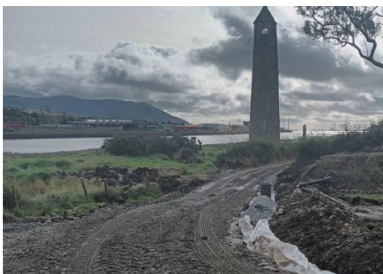
Earthworks adjacent to the Navigation Beacons
