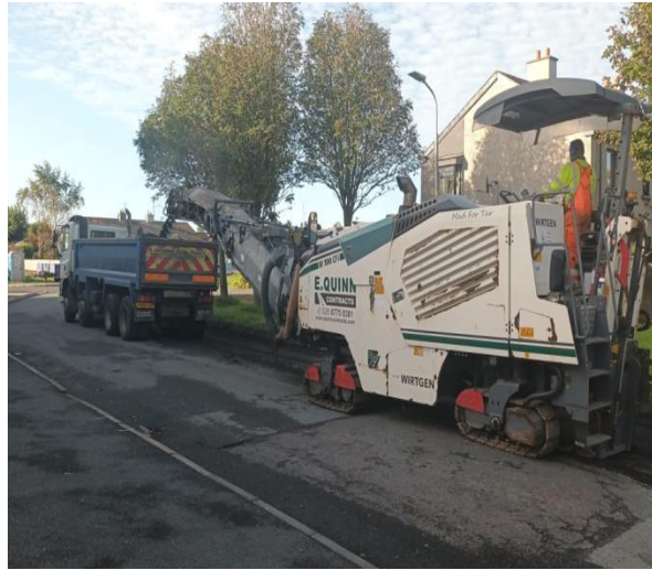
Plaining works at Aghameen Park, Dundalk
