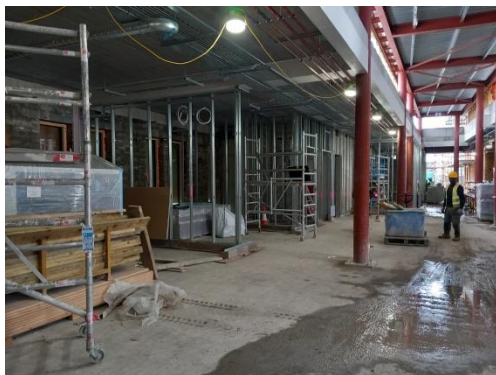
Block N New Link Building : Foyer (Reception) Area First Fix completed
