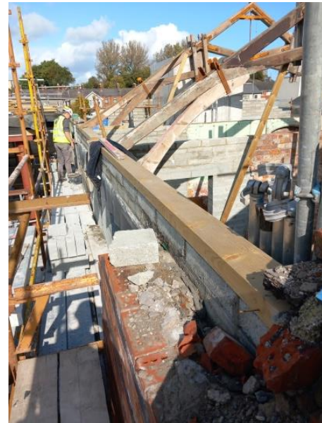
Block C West Room with Refurbished Trusses installed. Rafter install commenced, with felt and batten and slating to follow over the coming days
