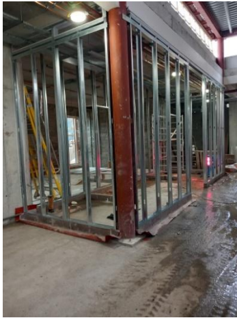
Block N: New Link Building internal walls fit out
