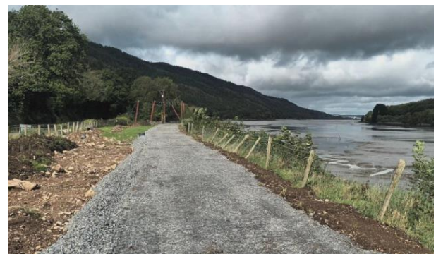
Sub base Placement
