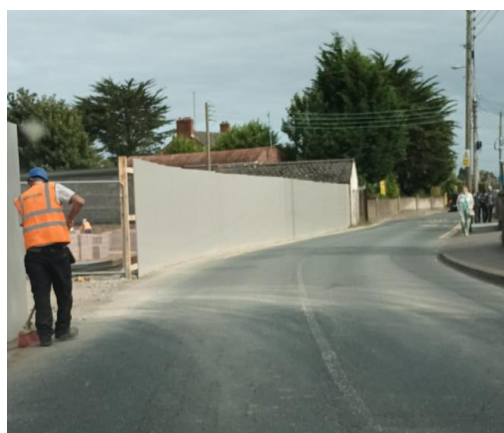
Works at Crushrod Avenue, Drogheda
