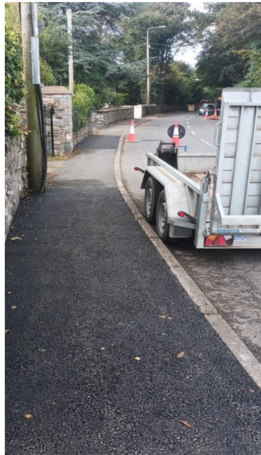
Footpath works at Point Road, Dundalk
