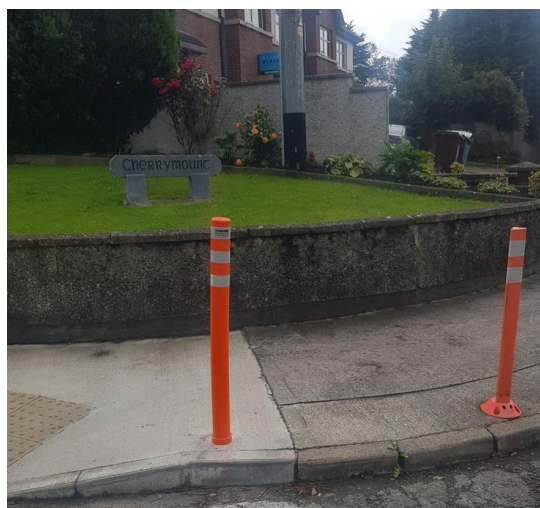
New bollards at Cherrymount
