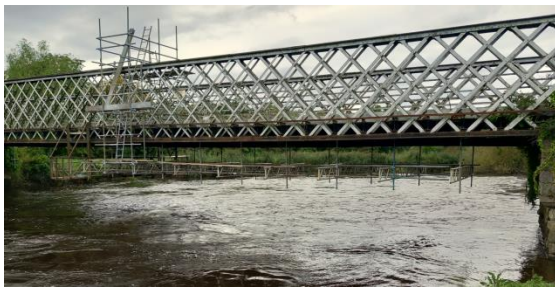
Encapsulation system commenced
