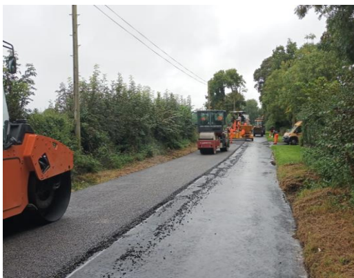
Roadworks at Tallanstown
