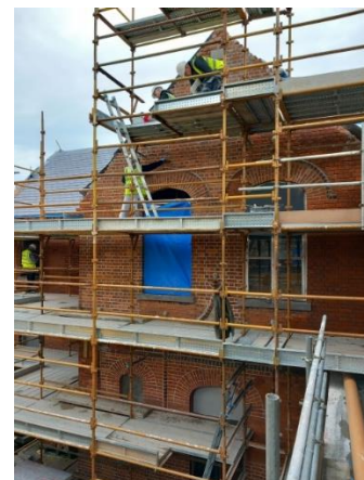
Lime Mortar repointing Block B
