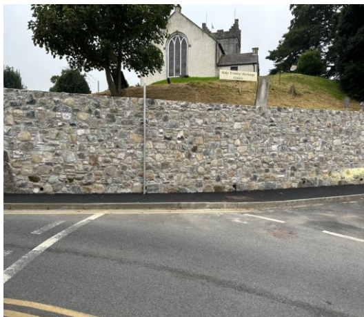
Repair of a boundary wall at the Heritage Centre in Carlingford
