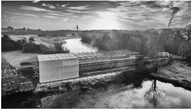
Drone footage of Bridge Encapsulation
