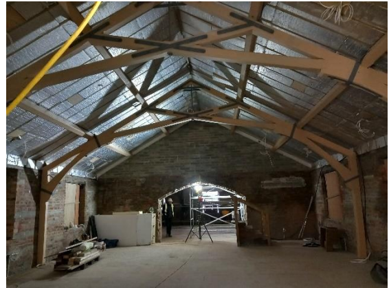
Block C Central Room with truss painting and ceiling insulation installation.
