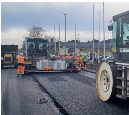
Roadworks at Monasterboice
