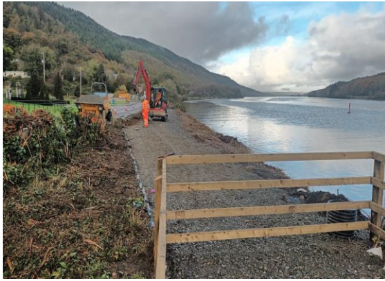
Cross-border section of CLG installed
