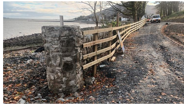
Seawall repairs through Omra Park
