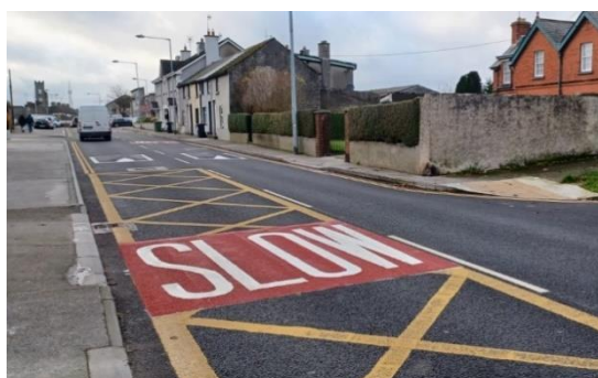
Low cost safety works at Scarlet Street (2)
