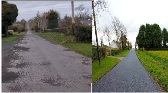
Roadworks at Funshog- Before & After
