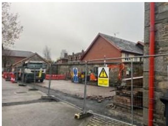
Construction works have commenced for the Varcities Project at the Open Space at the County Library
