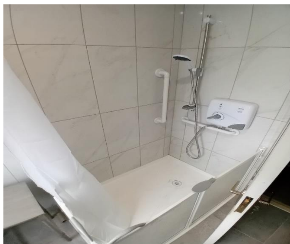
Bathroom Adaptation completed in Ardee in November, part funded with a Housing Grant for Disabled Persons
