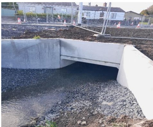
Culvert adjacent to Roundabout and council housing.
