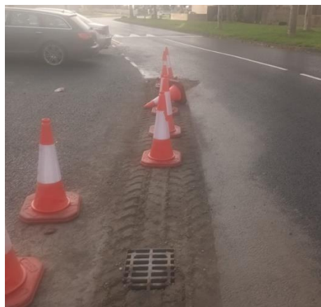
Drainage works in Muirhevnamor
