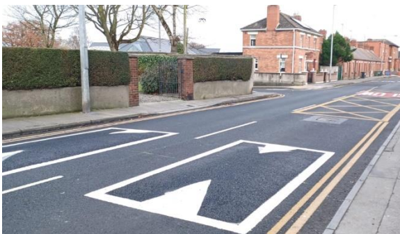
Low cost safety works at Scarlet Street
