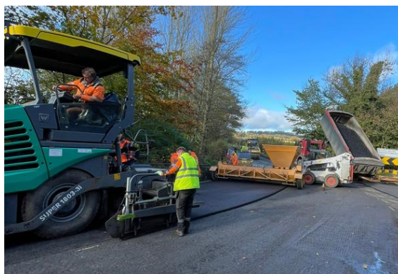
Roadworks at Nursery Cross, Collon
