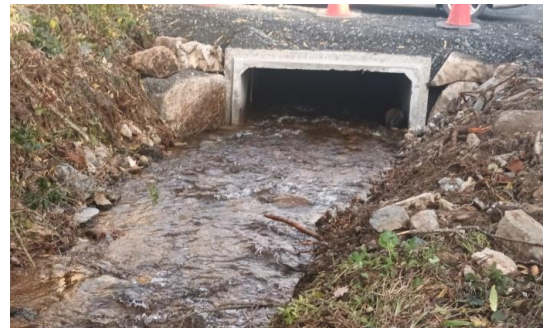
Culvert installation on Lower Shore Road
