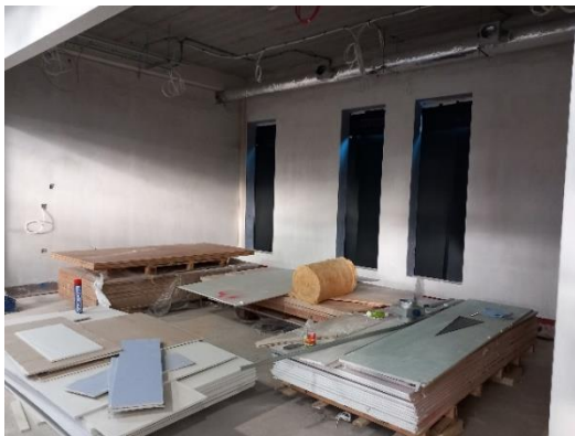
Block N New Link Building : Plastered Meeting Room 1
