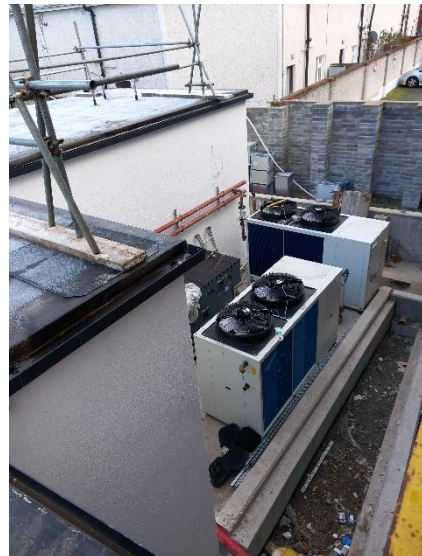
Block N: Mechanical Plant installation
