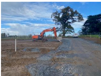
Access Road Construction
