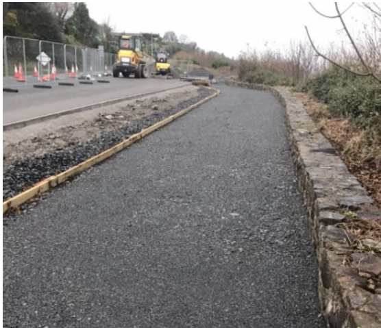
Works in Section 1 Carlingford
