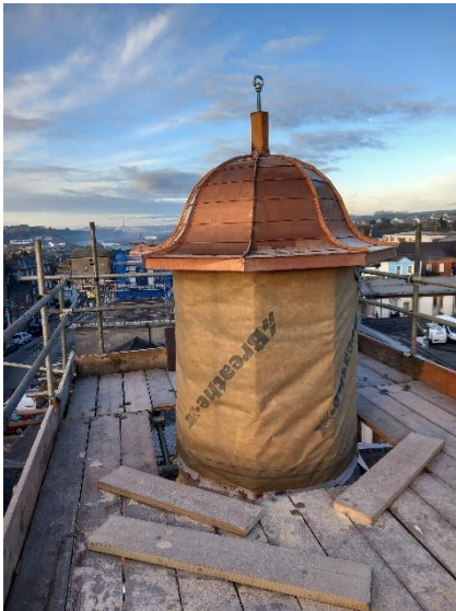
Block B Cupola installation
