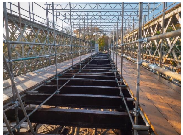
Obelisk Bridge Steel Support Beams after "flogging" by specialist contractors
