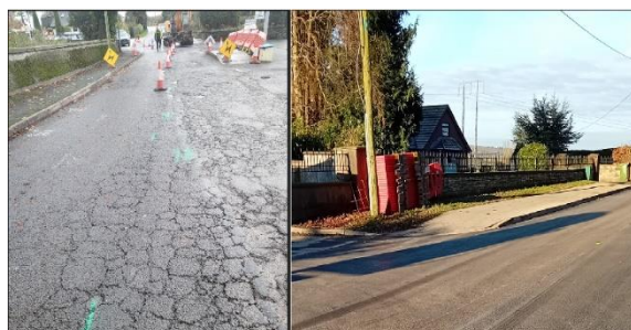
Roadworks at Tinure- Before & After
