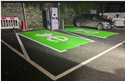
Works completed Ardee Car-park .
