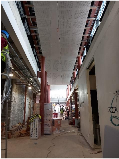
Block N New Link Building : Fit out
