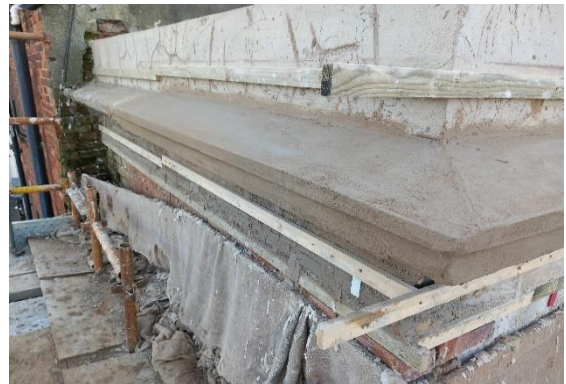
Block E Annex Building : Parapet Conservation Works
