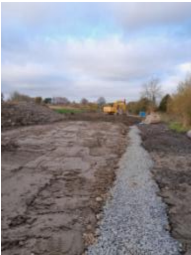
Backfilling of Pipeline
