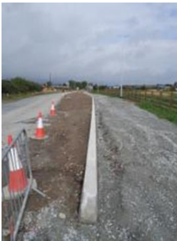
Footpath & Cyclelane Construction Progress
