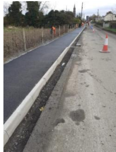
Stabannon Footpath- Works in Progress
