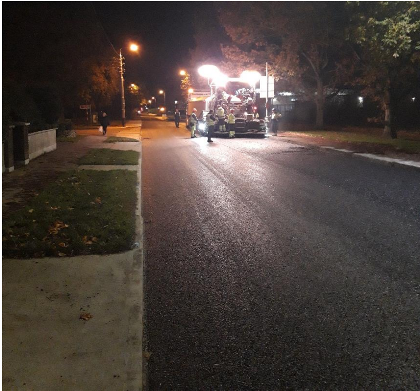
Road resurfacing works on the Ecco Road at night
