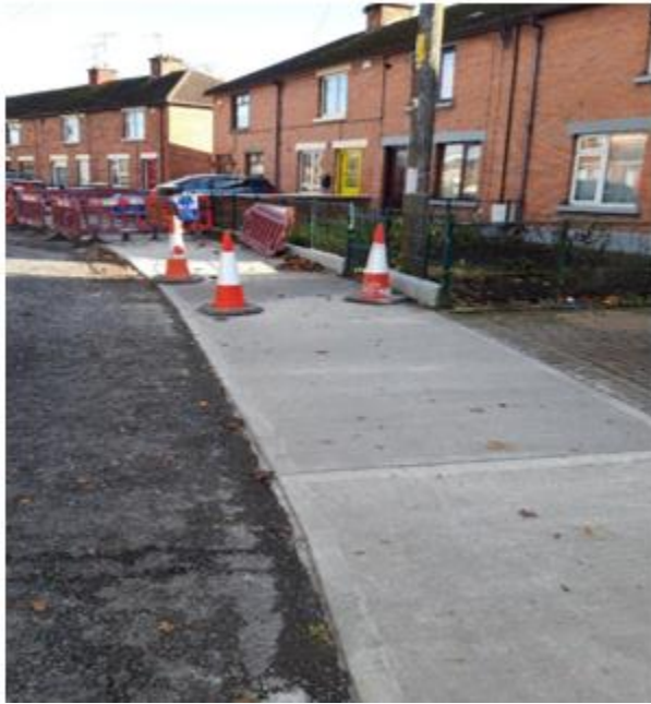
Footpath repairs at The Laurels Dundalk
