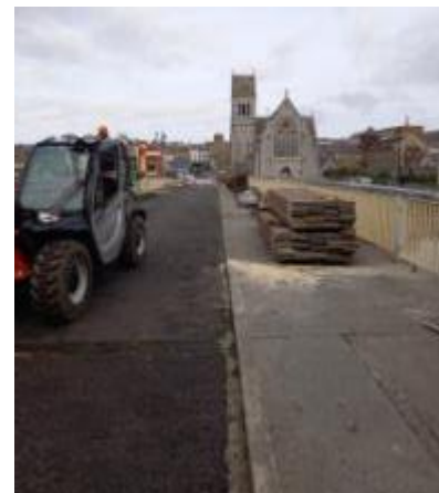
St Dominick's Bridge- Contractor setting up on site
