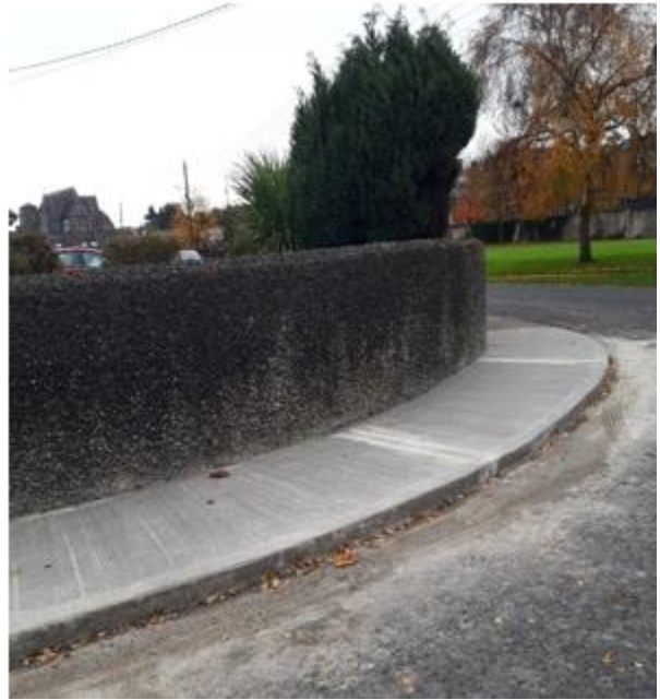
Footpath repairs at Pearse Park Dundalk
