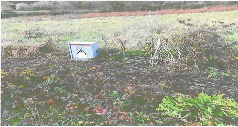
Site showing Electrical Panel Box (Picture 5)
