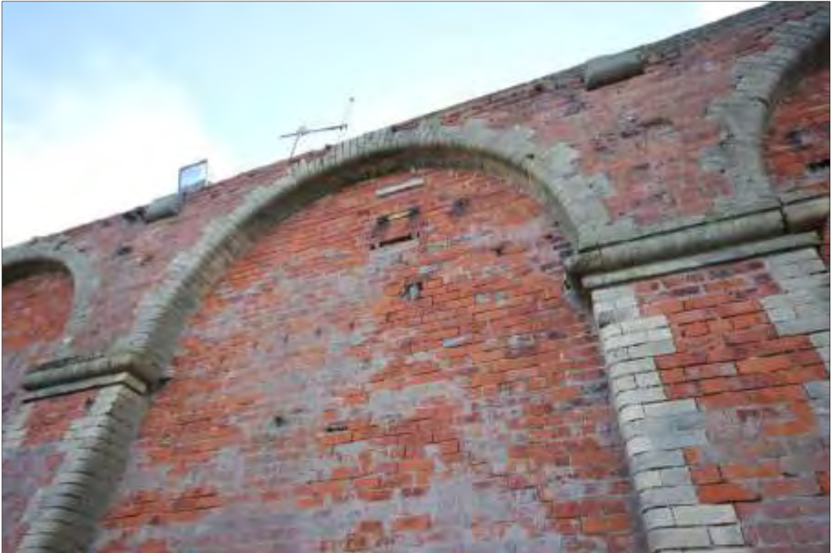
Plate 20: Close-up of arch to northwest elevation of redbrick wall
