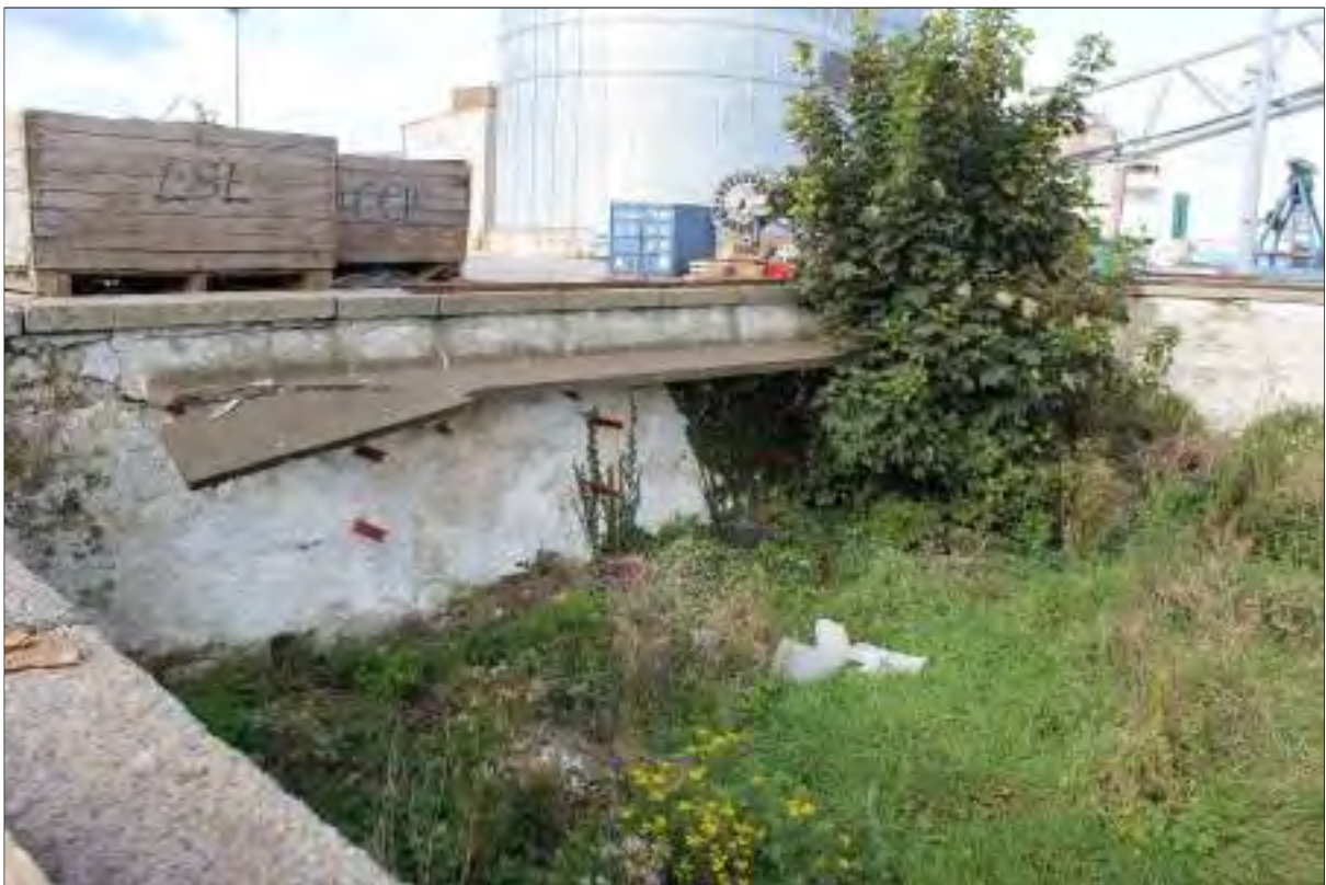
Plate 11: View of damaged ladder cover to wall surrounds of lighthouse and keeper's house, facing west
