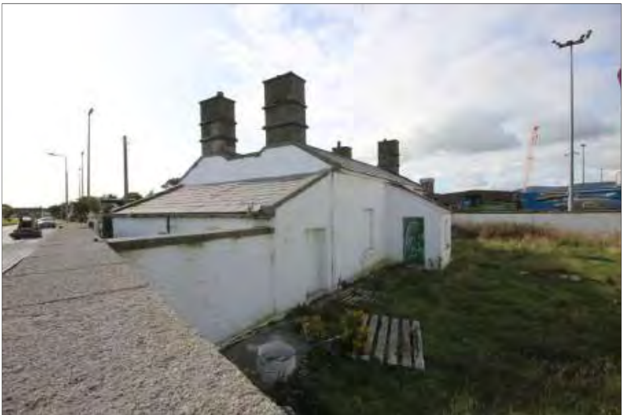
Plate 13: View of keeper's house, facing south-southwest
