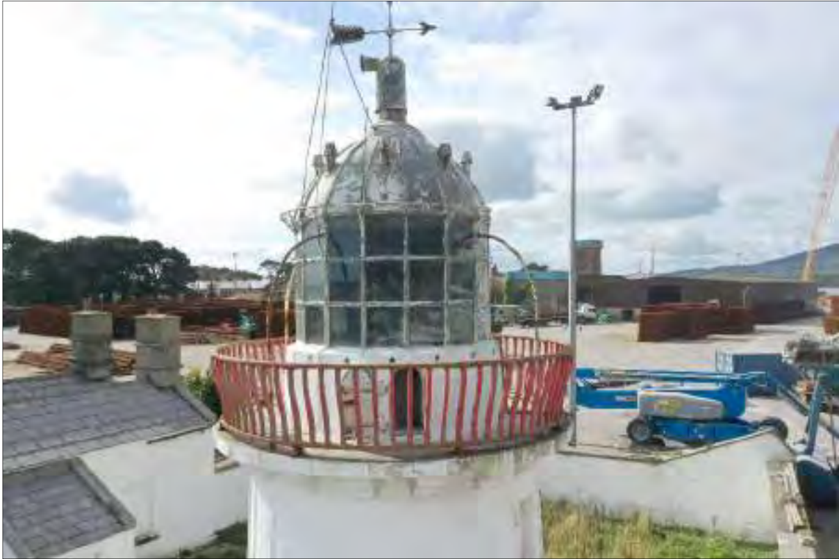
Plate 8: Aerial view of lighthouse showing first floor door, facing south-southwest
