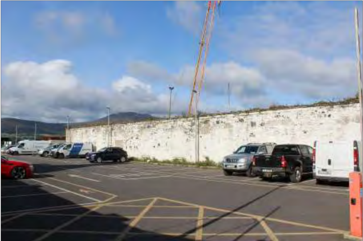
Plate 28: View of southeast elevation of wall proposed for removal, facing west-northwest
