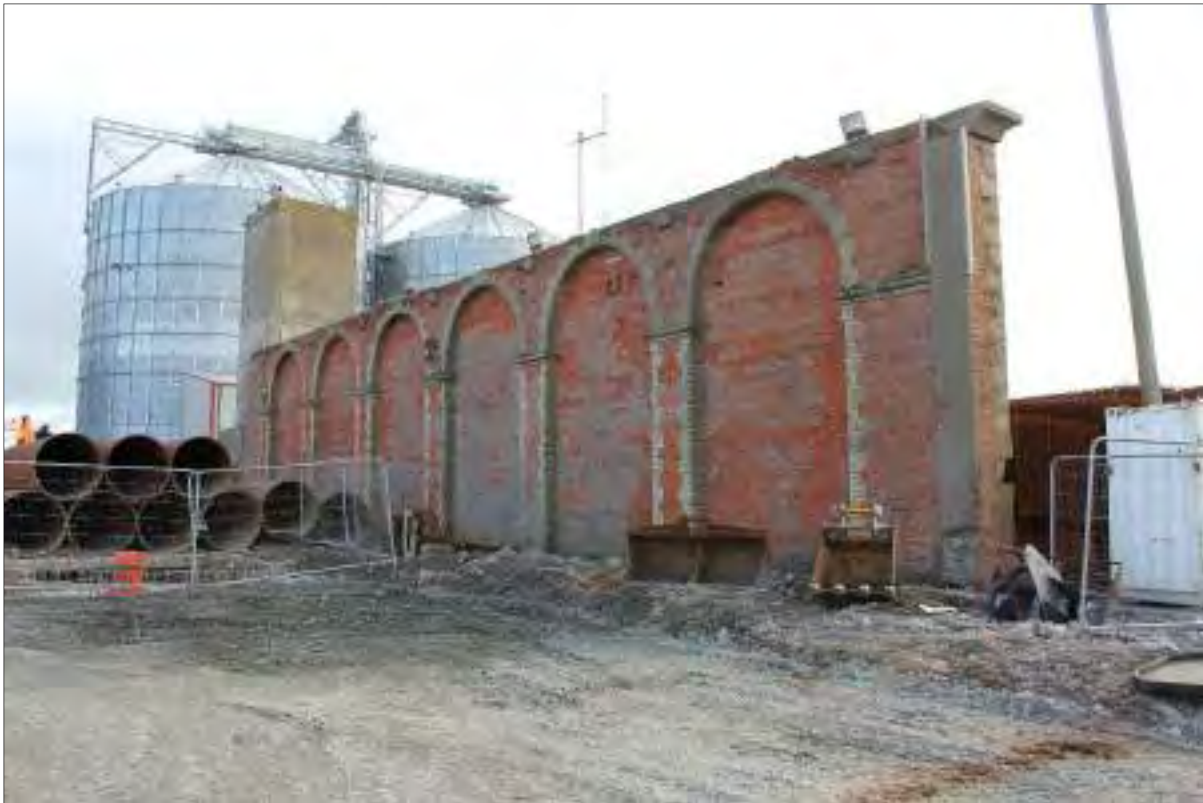
Figure 11: View of northwest elevation of redbrick wall, facing northeast
