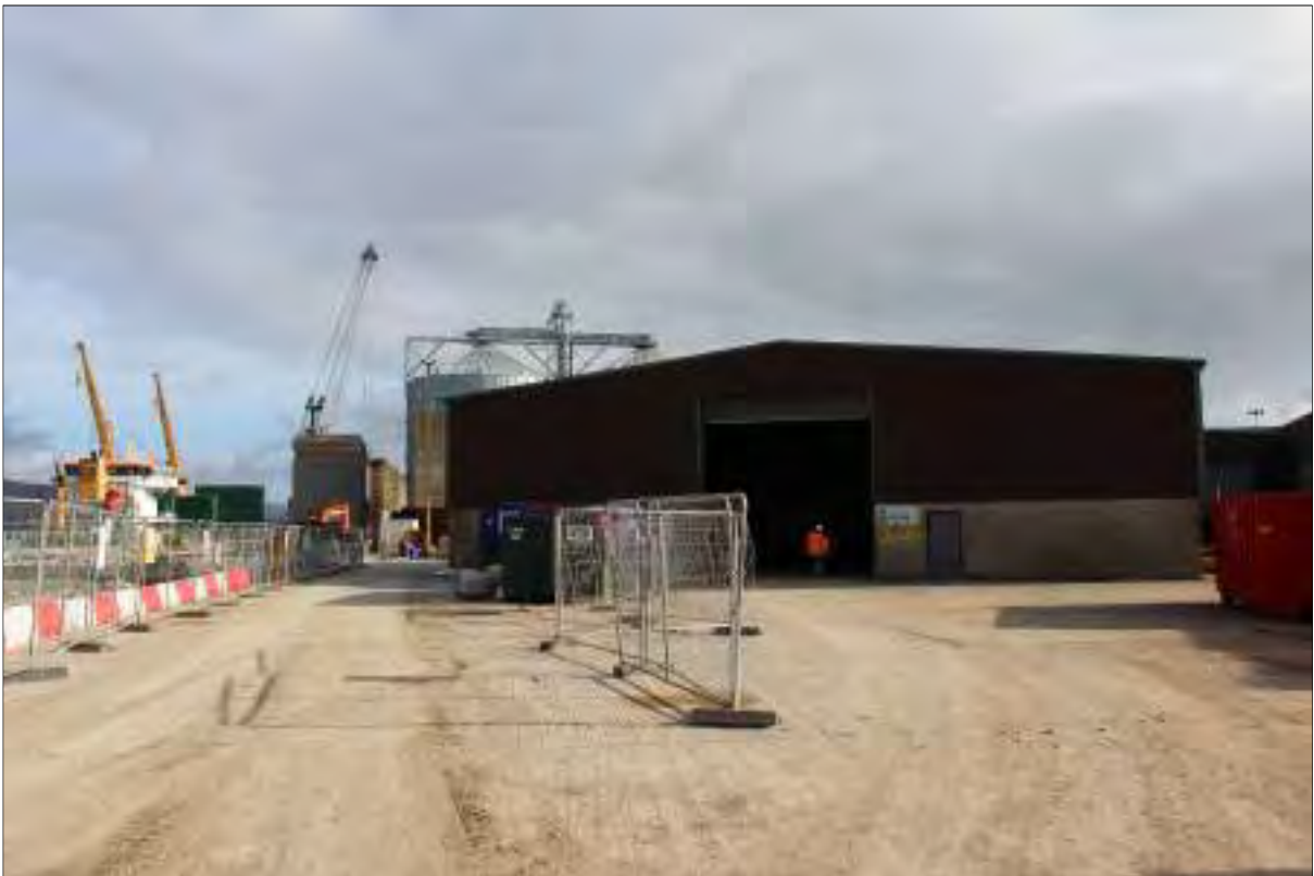
Plate 25: View of building proposed for extension, facing northeast
