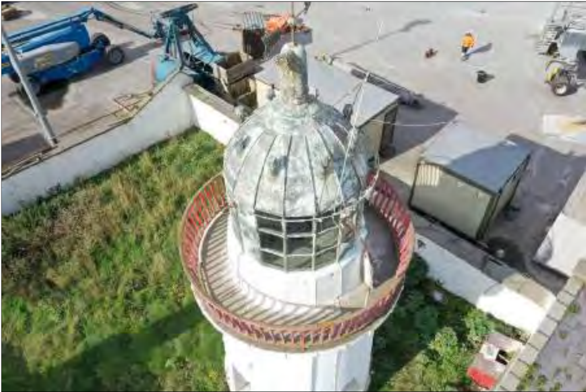
Plate 7: Aerial view of lighthouse, facing northwest
