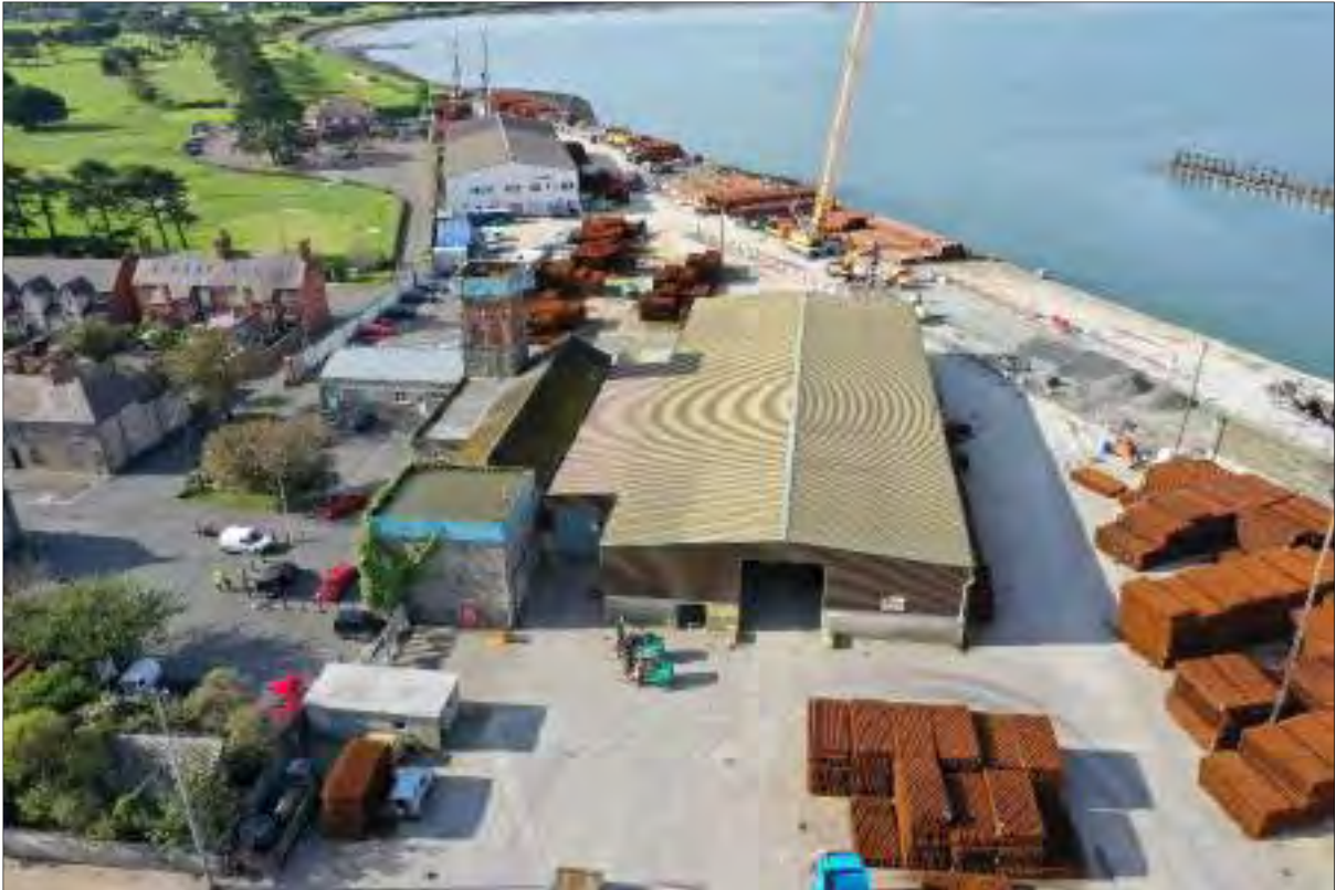
Plate 24: Aerial view of building proposed for extension, facing southwest
