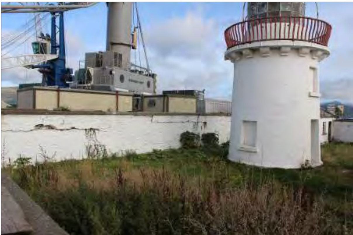
Plate 9: View of damaged wall surrounds of lighthouse and keeper's house, facing north
