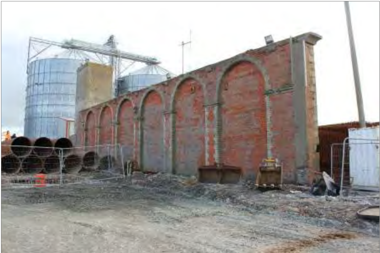
Plate 18: View of northwest elevation of redbrick wall, facing northeast
