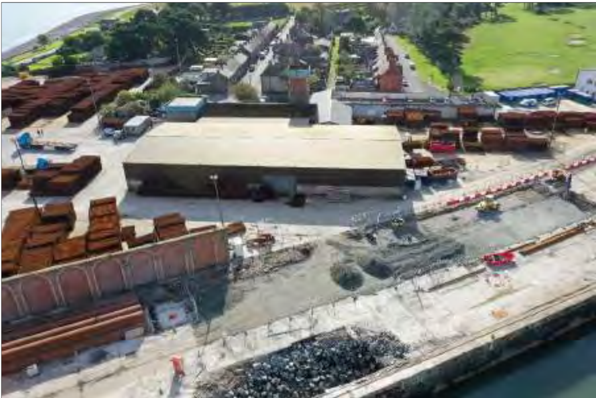
Plate 23: Aerial view of building proposed for extension, facing southeast
