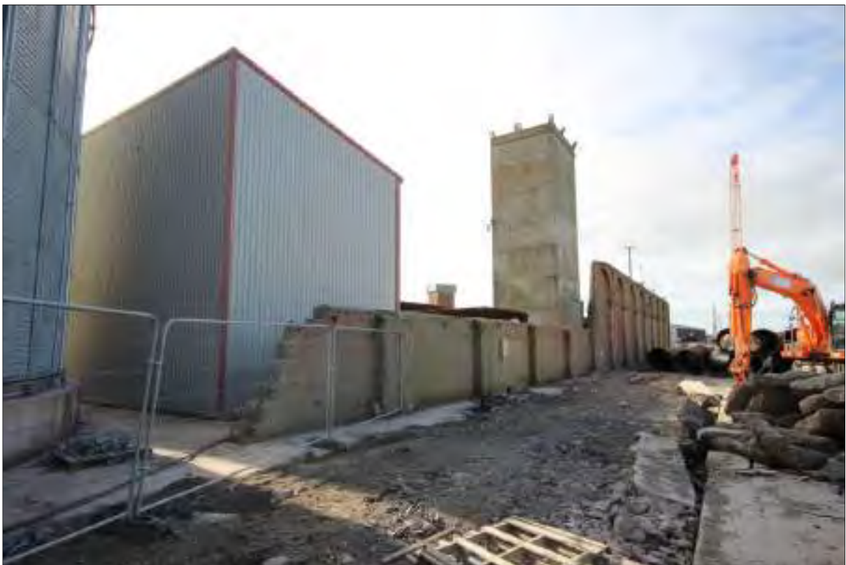
Plate 19: View of northwest elevation of redbrick wall, facing south-southwest
