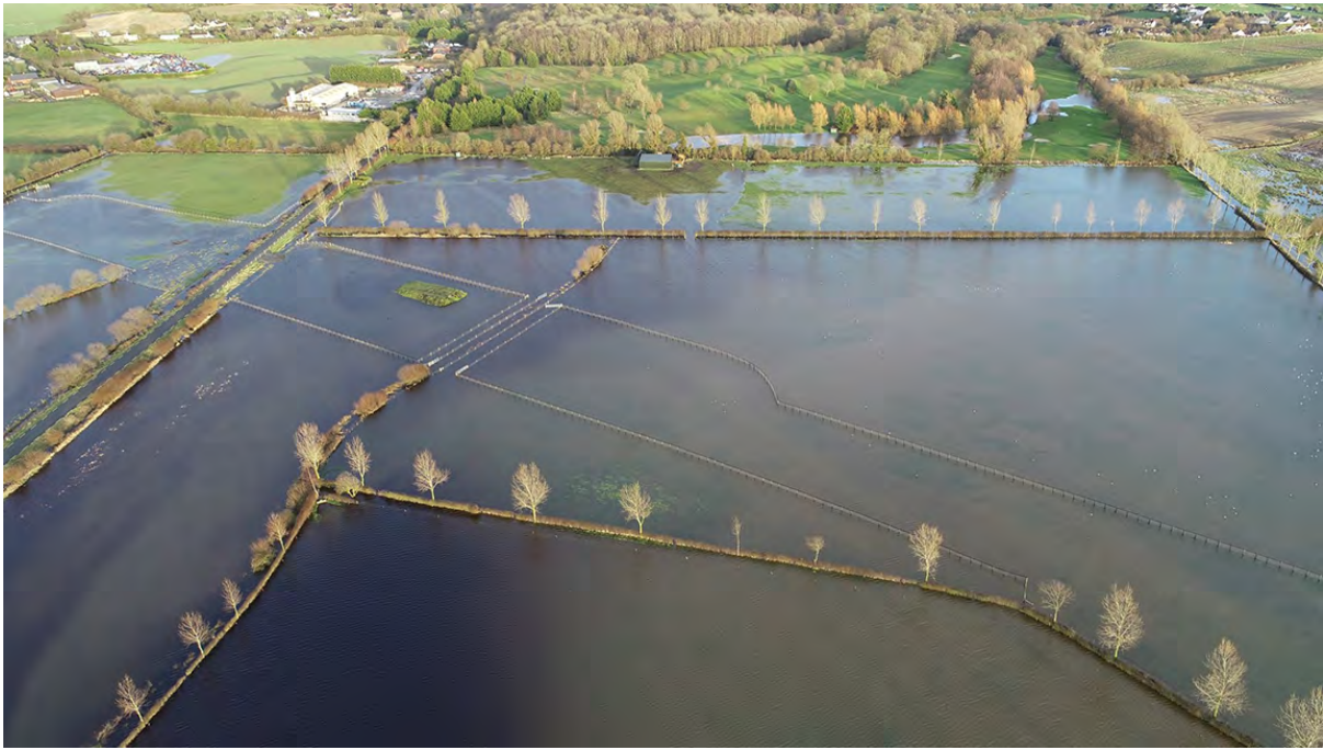
Fencing for the N52 Ardee Bypass clearly visible in Ardee Bog floodwaters. The fencing was illegally installed in November 2019 after all work on the N52 Ardee Bypass was ordered to cease by the Oireachtas. Photo: Seán Walsh, February 25, 2020.
